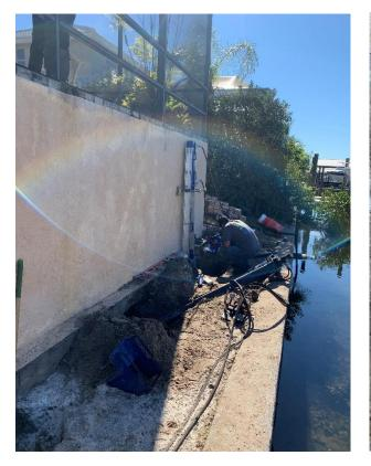
that connected to an all-threaded rod. SafeBase<sup>™</sup> Push Piers were then installed inline with the helical tiebacks and the pier bracket adapter was installed to restrain the SaberTooth<sup>™</sup> Push Pier bracket. With the helical piers and push piers in place the footing can longer settle or slide away from the home towards the water. A total of eight helical tiebacks and push piers were installed in February of 2022.
