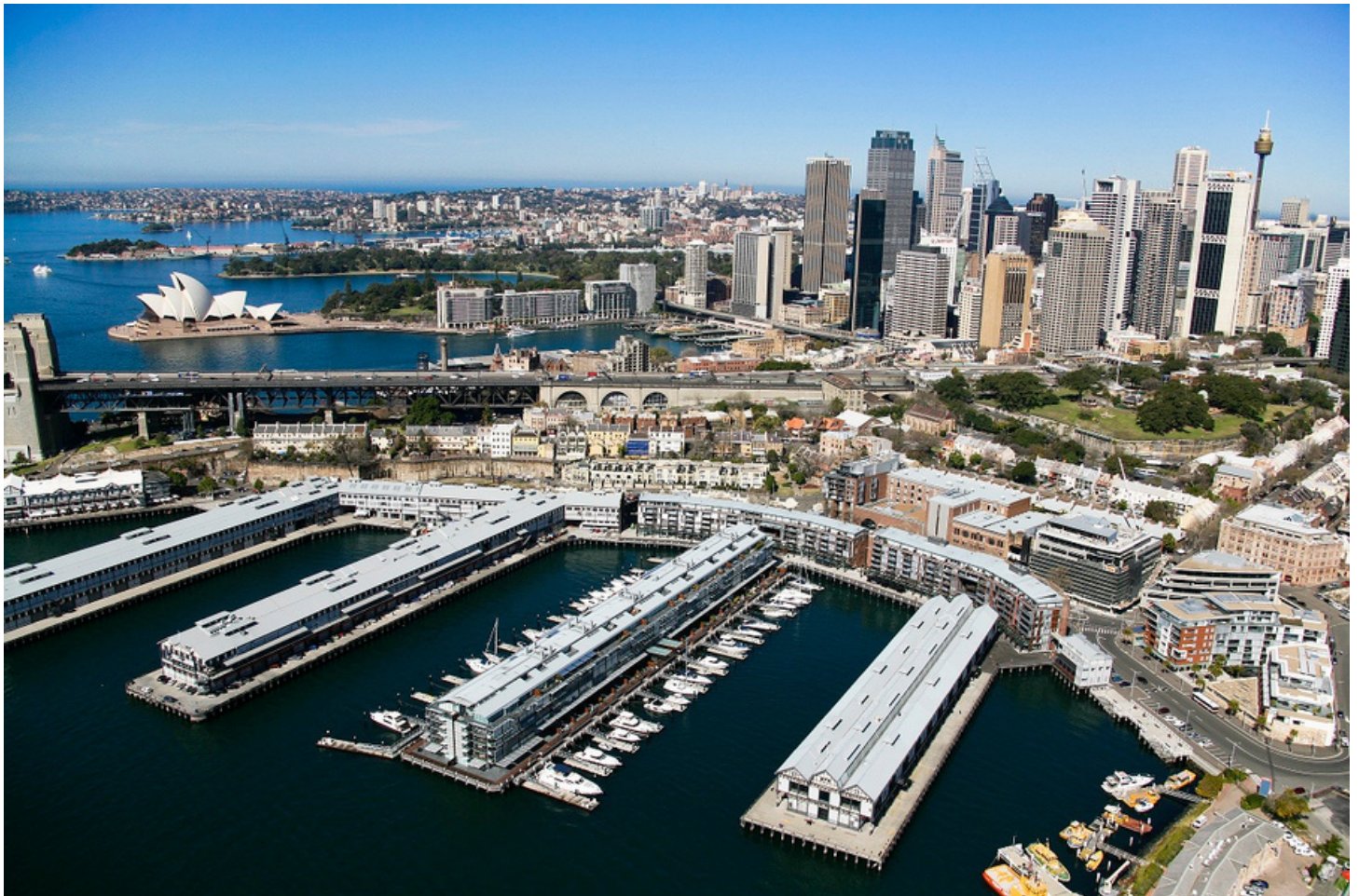
Piers 8/9 Walsh Bay, Sydney
