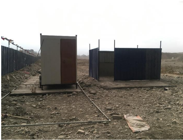
Photo Clip 7: Toilets and bath rooms at site
