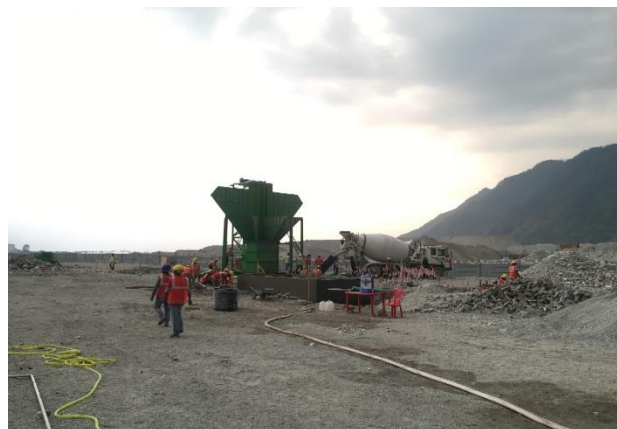
Photo clip 9: Erection of Batching Plant in progress, Workers using PPE
