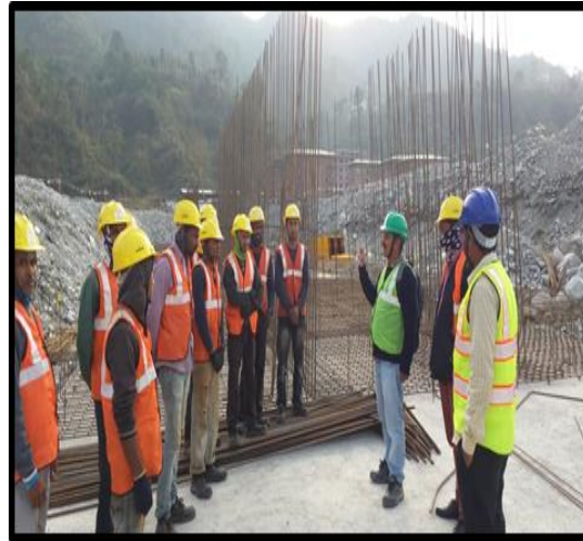
Tool box talk at outfall No.3
