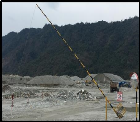
Drop gate to restrict unauthorized vehicle entry
