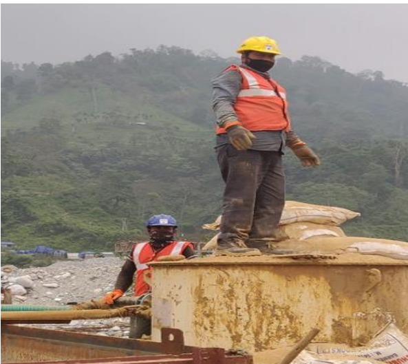
Worker in proper PPE gear
