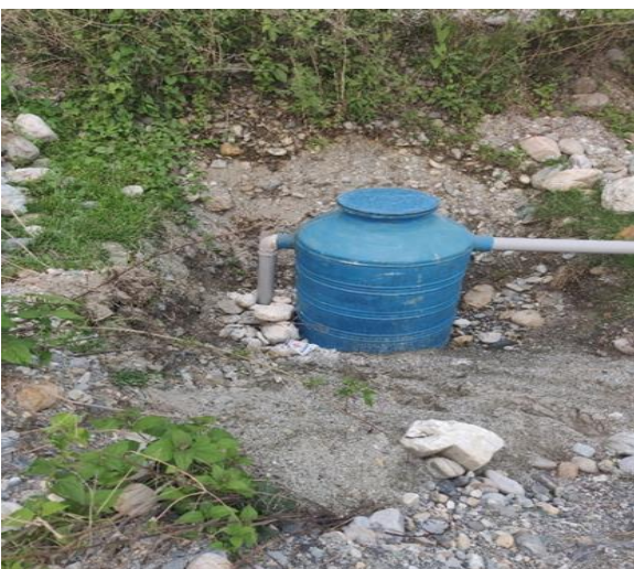
Sealed sewage tank opening to avoid odor and soil contamination
