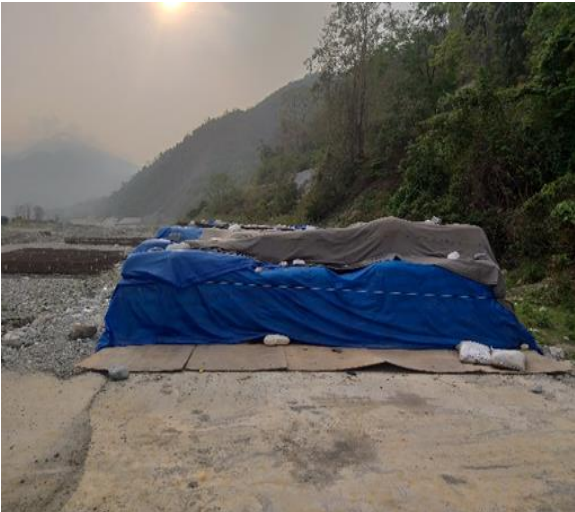
Bentonite sacks covered in Tarpaulin sheet and barricaded
