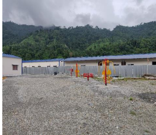
Workout equipments installed at workers camps
