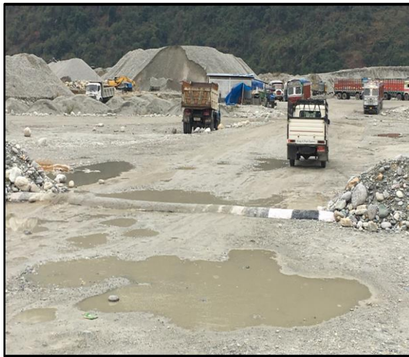
Speed Breaker between Camp and Lay down Area
