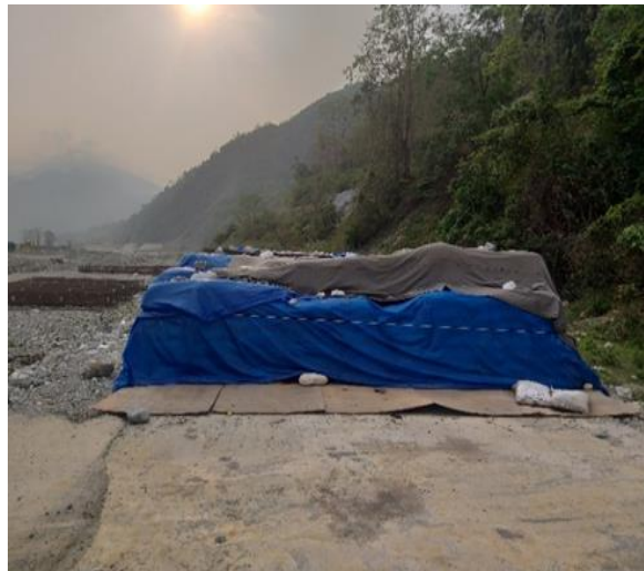
Now: Bentonite sacks removed from the well barricaded pile.
