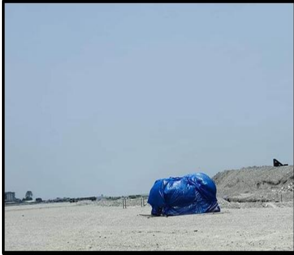
Preventative measures taken in earthwork area
