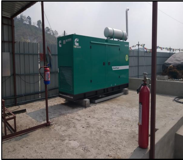
Fire Extinguishers at the DG and Switch yard Area
