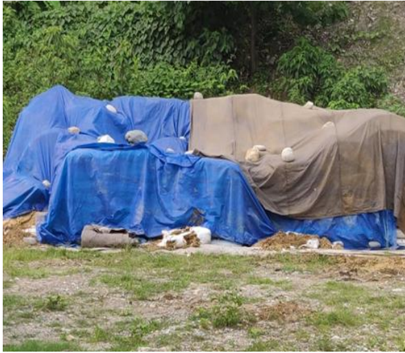
Before: Bentonite sack around site covered and well barricaded
