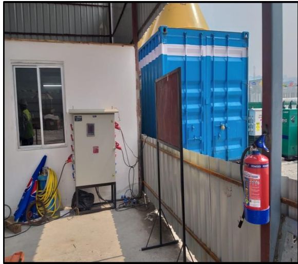
Fire Extinguisher at the workshop
