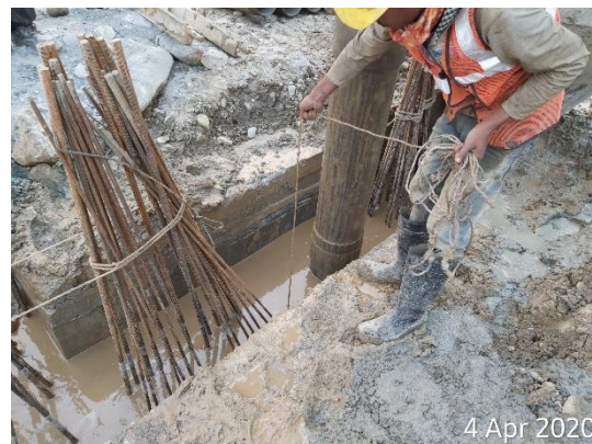
Concrete finish level check
