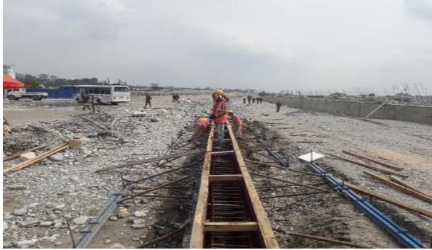
Rebar arrangement and alignment check
