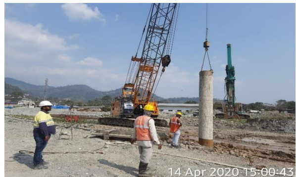
Stop end installation
