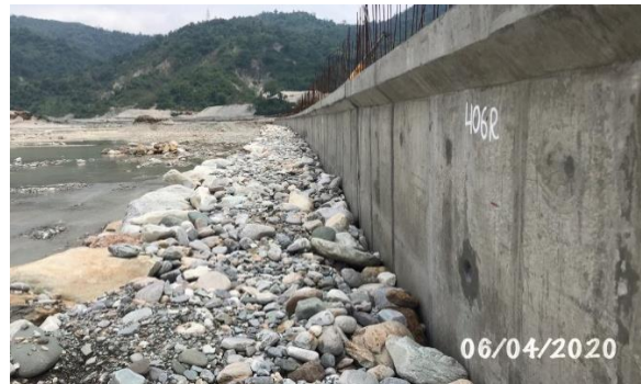
Concreted panel of cast in situ wall
