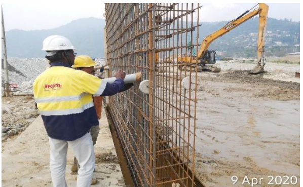
Rebar cage and weep holes installation
