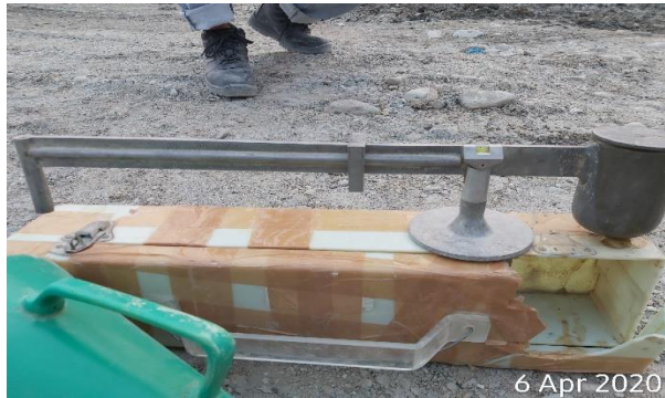
Bentonite density test
