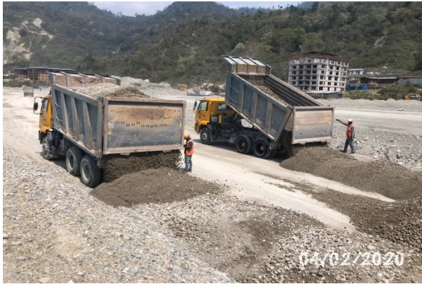
Dumping and Spreading for earth filling work
