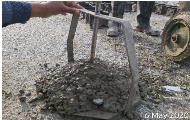
Slump test for Cast-in-situ wall
