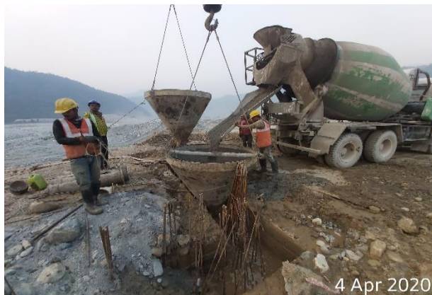
Concreting the D-Wall panel
