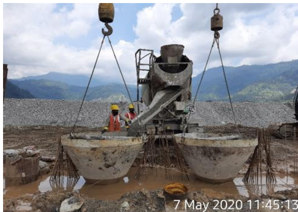
Concreting the D-Wall panel
