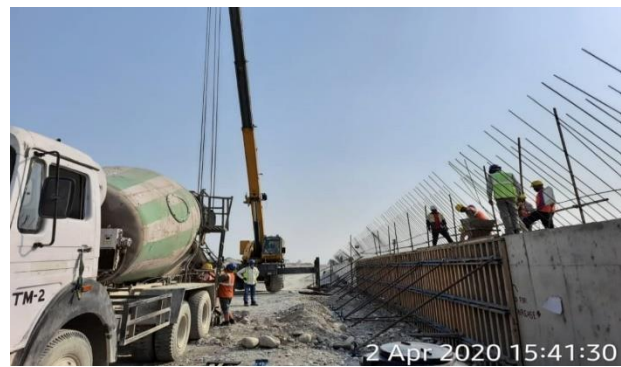
Concreting and compaction of concrete for cast-in situ
