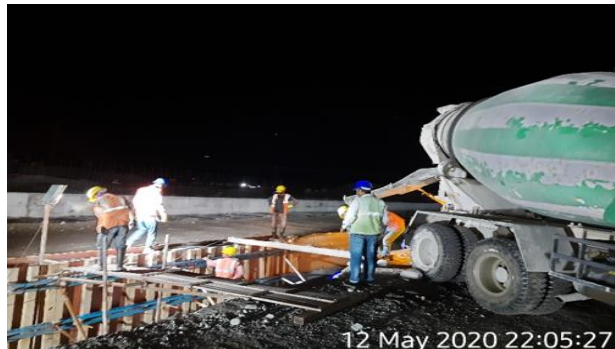
Slump test and concreting for dead man anchor blocks
