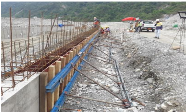
Rebar arrangement and alignment check
