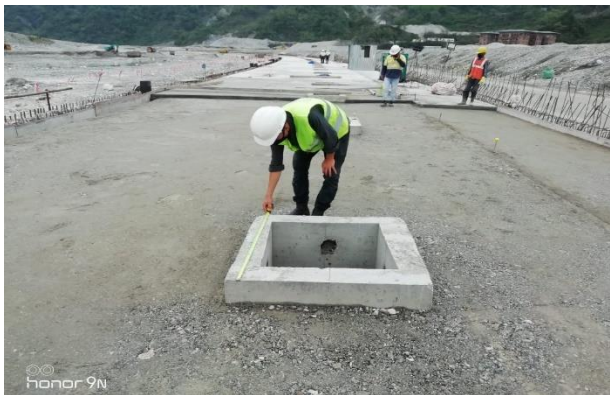
After installing Tree pit at Lower walkway
