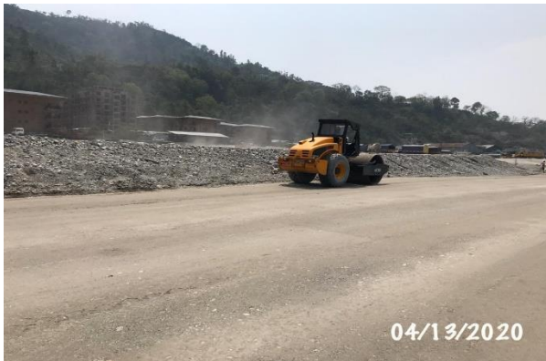
Compacting the earth fill
