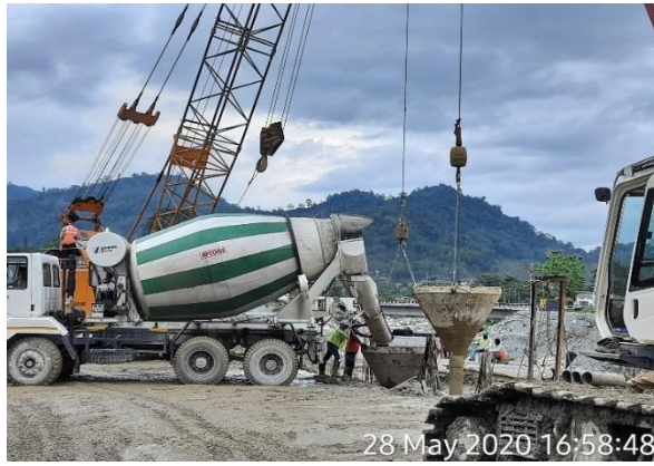
Concreting the D-wall panel
