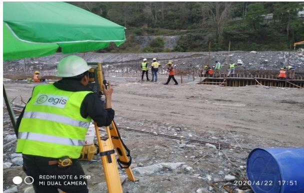
Rebar and alignment check
