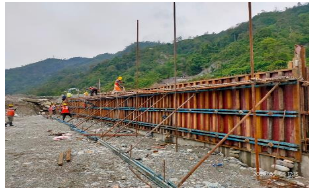
Formwork and reinforcement installations
