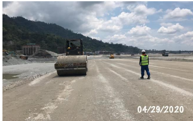
Compacting the earth fill
