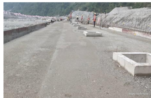
After installing Tree pit at Lower walkway
