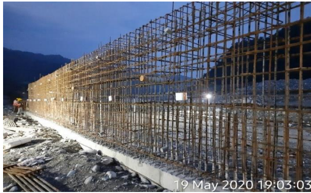
Formwork and reinforcement installations
