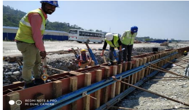
Rebar arrangement and alignment check
