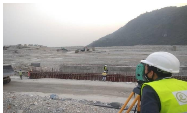
Rebar arrangement and alignment check
