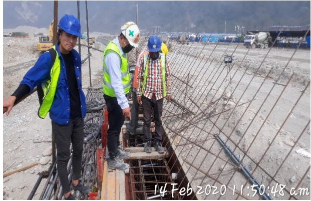
Formwork and reinforcement installations
