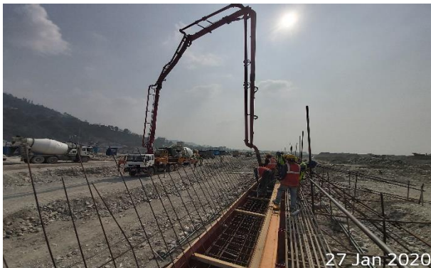
Concreting and compaction of concrete for cast-in situ
