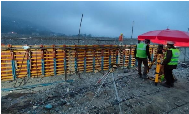
Rebar level check
