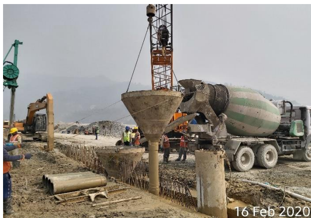
Concreting the D-Wall panel
