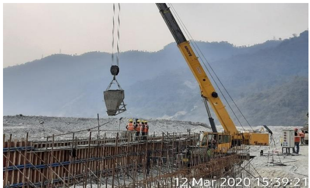
Concreting and compaction of concrete for cast-in situ
