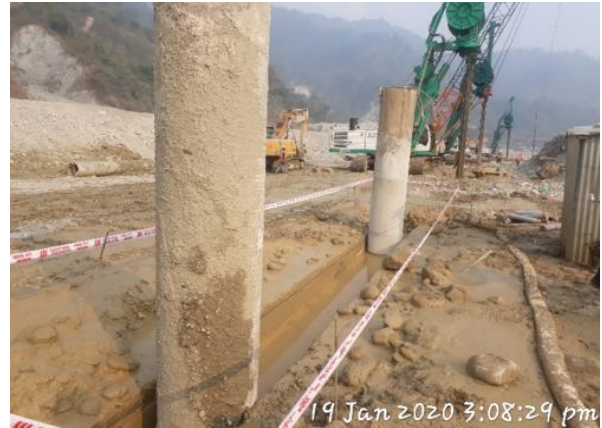
Stop end installation
