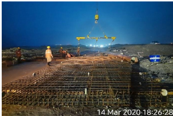
Rebar cage and weep holes installation
