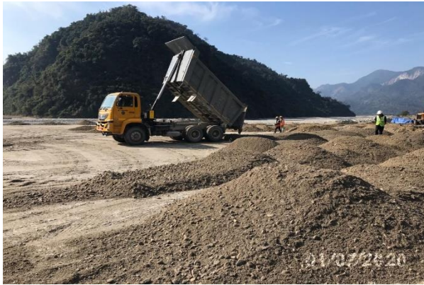
Dumping and Spreading for earth filling work
