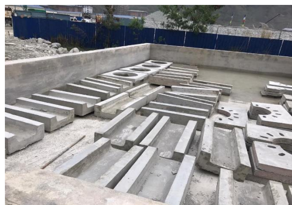
Precast of channels
