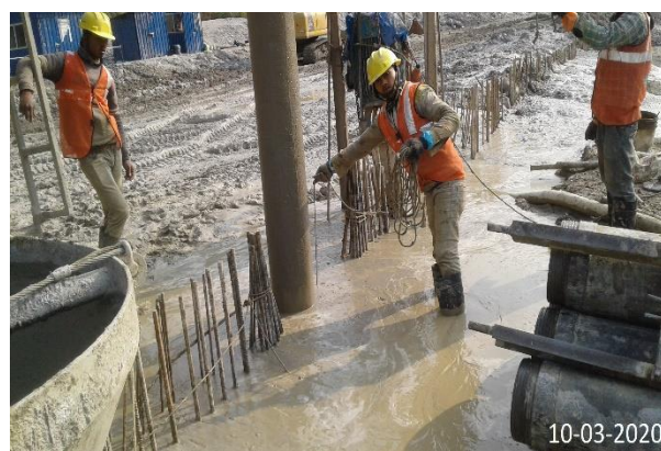
Concrete finish level check
