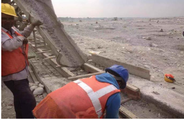
Guide wall: Top flange concreting
