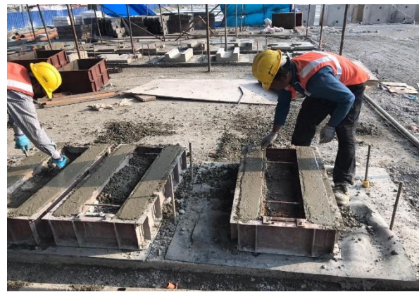
Precast of channels
