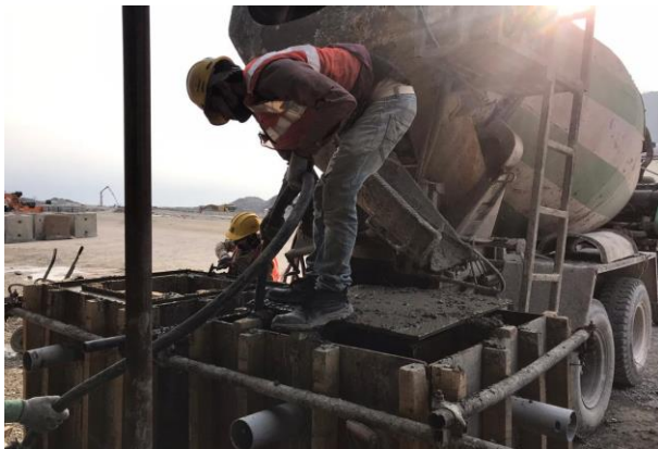
Concreting and curing for tree pits
