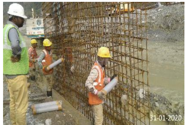
Rebar cage and weep holes installation
