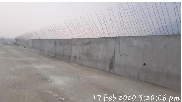
Concreted panel of cast in situ wall
