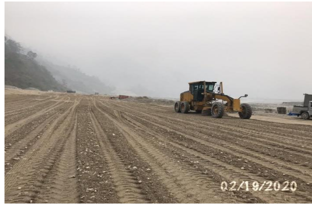
Dumping and Spreading for earth filling work
