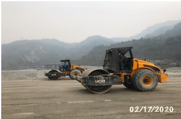
Compacting the earth fill
