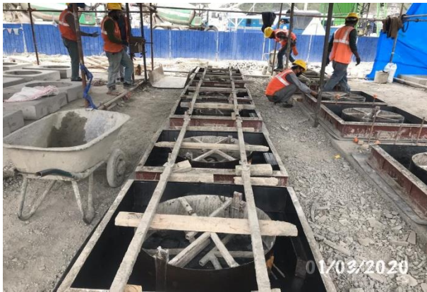
Mould preparation and concreting of grass paver blocks
