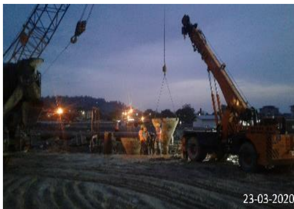
Concreting the D-Wall panel
