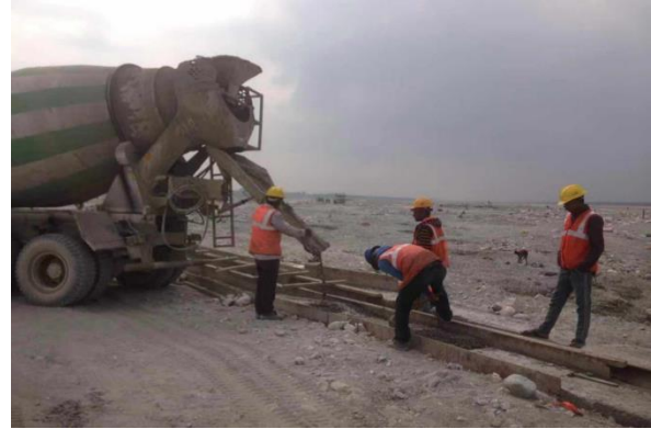
Guide wall: Top flange concreting
