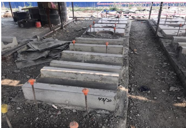
Precast of channels
