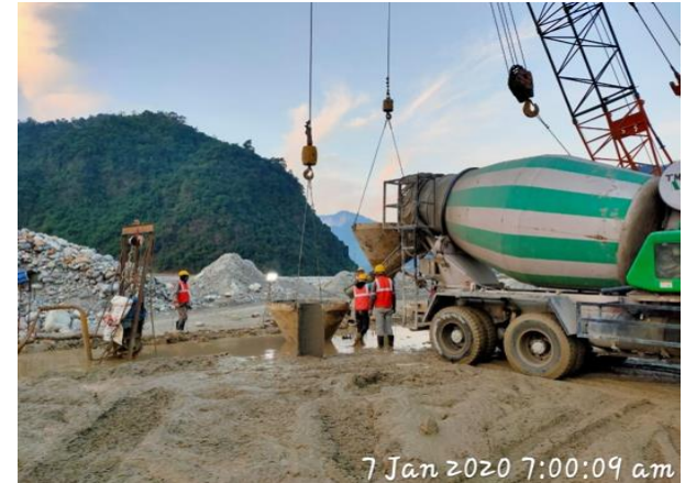
Concreting the D-wall panel
