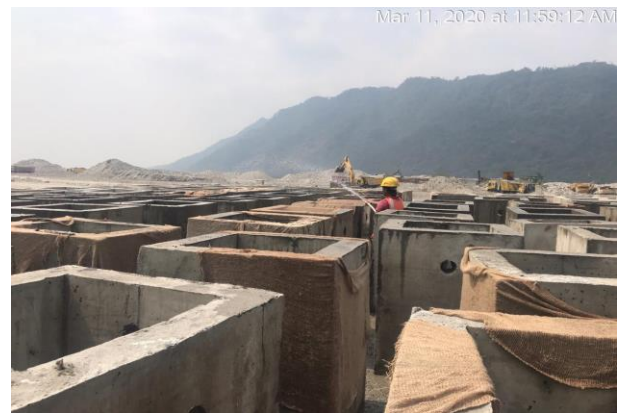
Concreting and curing for tree pits
