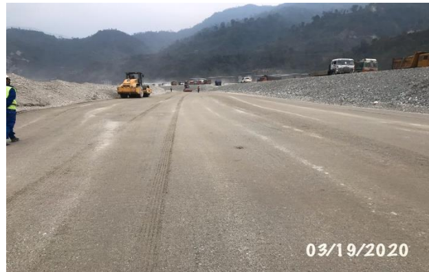
Compacting the earth fill
