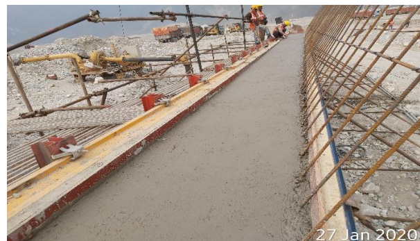
Concreted panel of cast in situ wall
