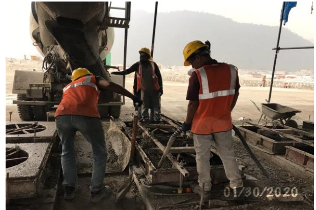
Mould preparation and concreting of grass paver blocks
