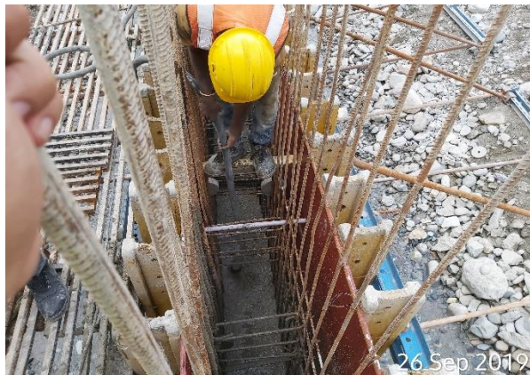
Using vibrator for concrete compaction
