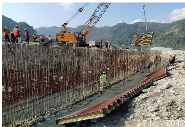
7 Nov 2019 Rebar arrangement and level check for cast in situ wall
