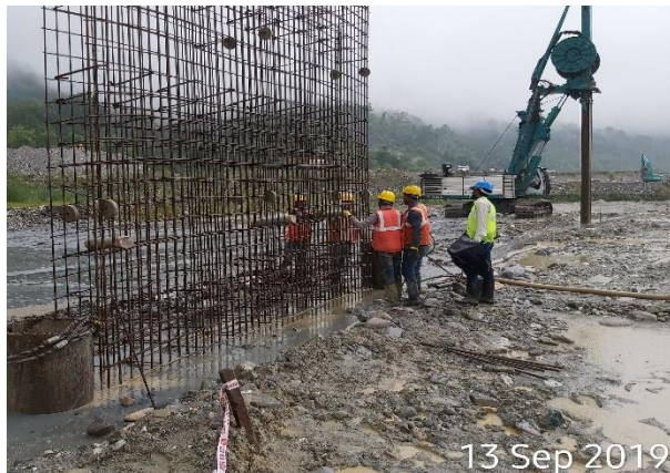
Rebar cage installations
