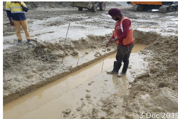
Sounding check after excavation works
