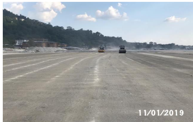
Compacting the earth fill
