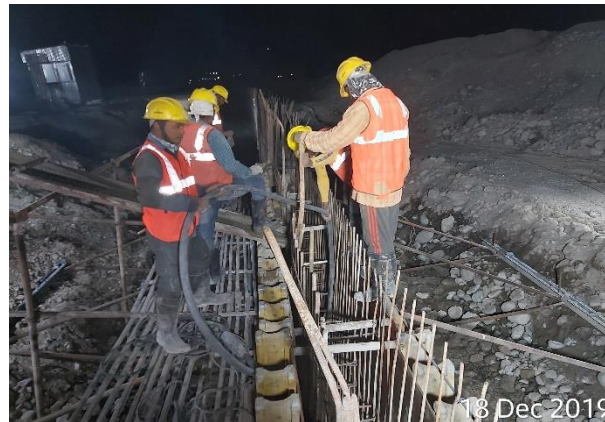
Using vibrator for concrete compaction
