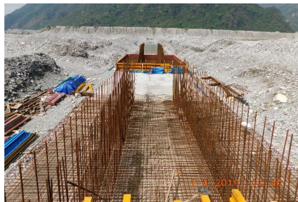
Reinforcement preparations for the open portion of outfall
