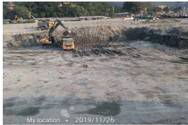
Removal of unsuitable materials before earth filling work
