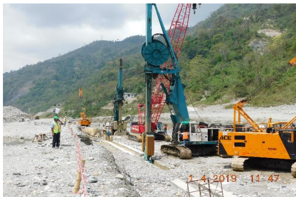
Diaphragm wall excavation works
