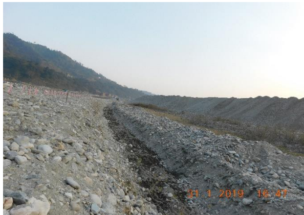
Guide wall work: Excavations and formwork preparations for vertical wall
