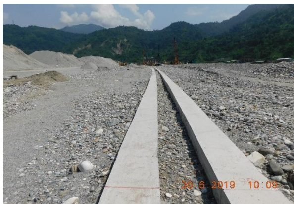
Guide wall concreted
