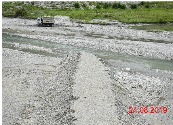
Spurs at end termination at PART-8
