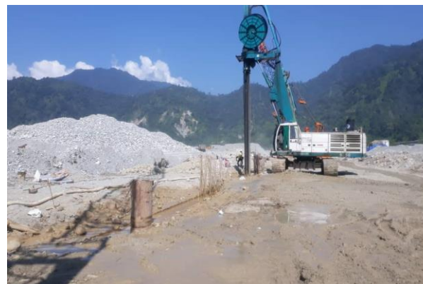
Diaphragm wall excavation works
