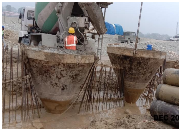
Concreting the Diaphragm wall panel
