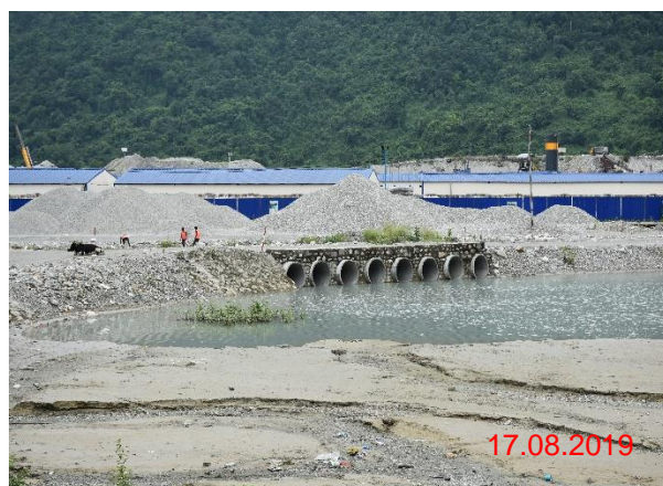
Hume pipe above the Staff quarter and below the NHDCL colony
