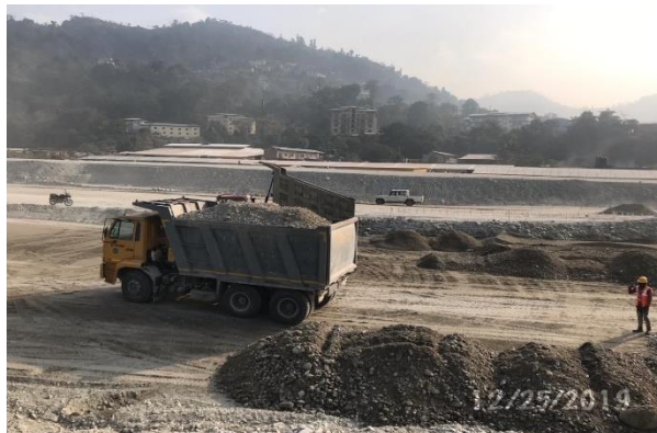
Dumping and Spreading for earth filling work
