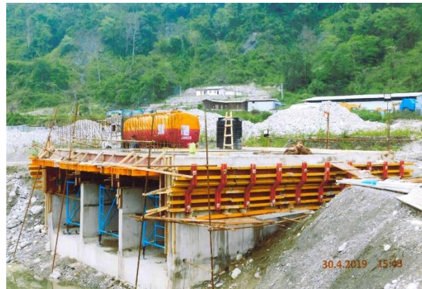
Reinforcement arrangements, concreting and formworks for ducted portion
