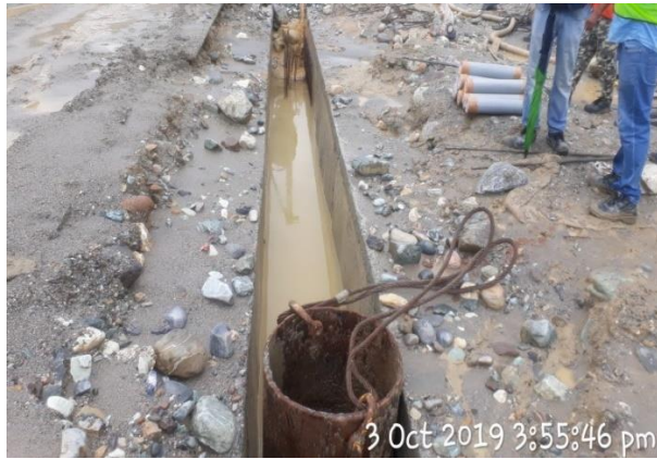
Stop end installation
