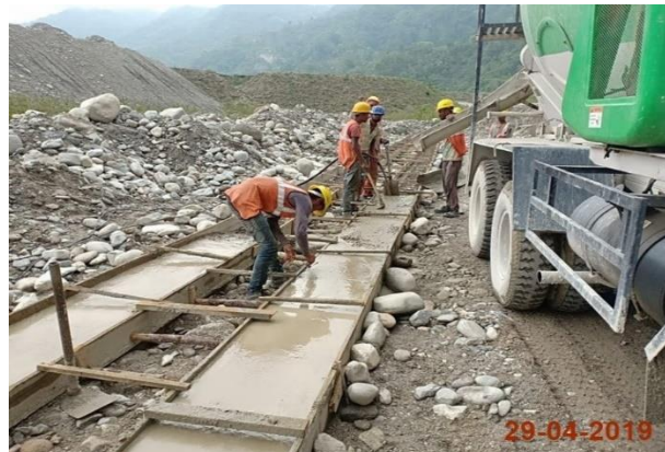
Guide wall work: Formwork and concreting for the top flange
