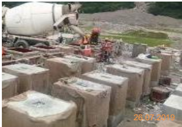
Curing the blocks at site
