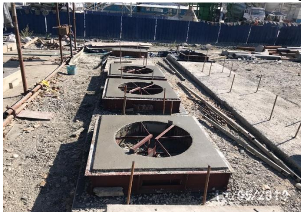
Removal of formworks
