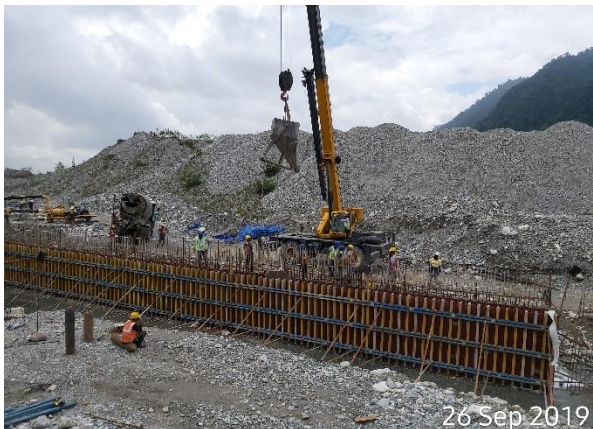
Concreting the cast in-situ wall panel
