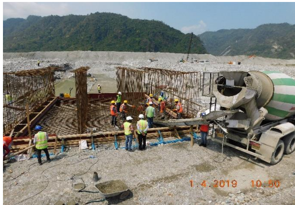
Reinforcement arrangements, concreting and formworks for ducted portion
