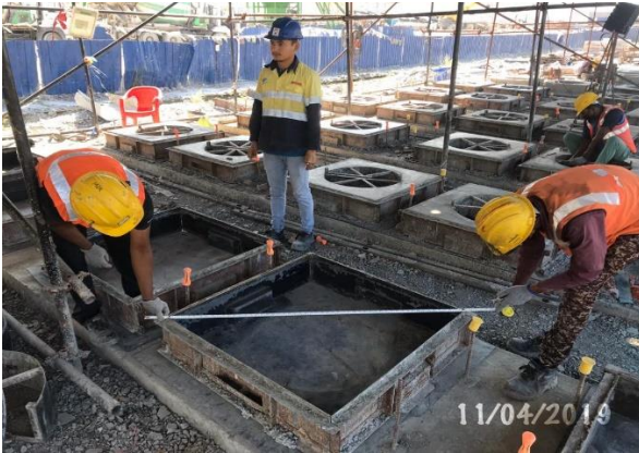
Formwork preparation for precast blocks
