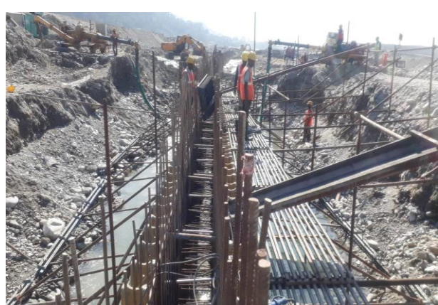
Concreting the cast in-situ wall panel
