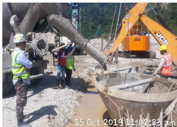
Concreting the Diaphragm wall panel
