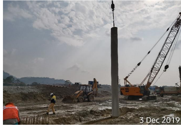
Stop end installation
