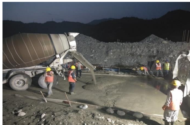
Excavations and PCC laying for the outfall structures
