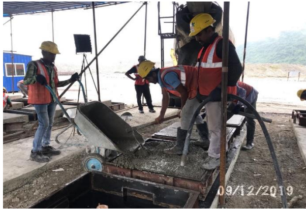
Using vibrators for compaction of concrete
