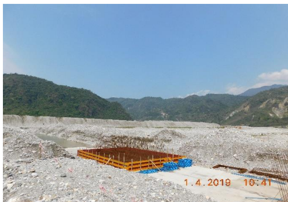
Reinforcement preparations for the open portion of outfall
