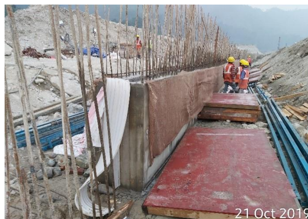
Removal of formwork for concreted panel of cast in-situ wall
