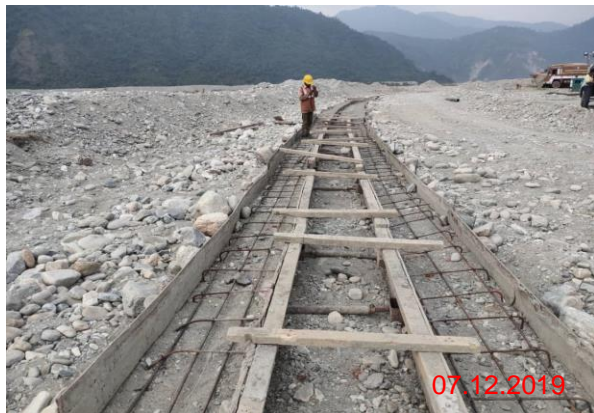
Guide wall work: Formwork and concreting for the top flange
