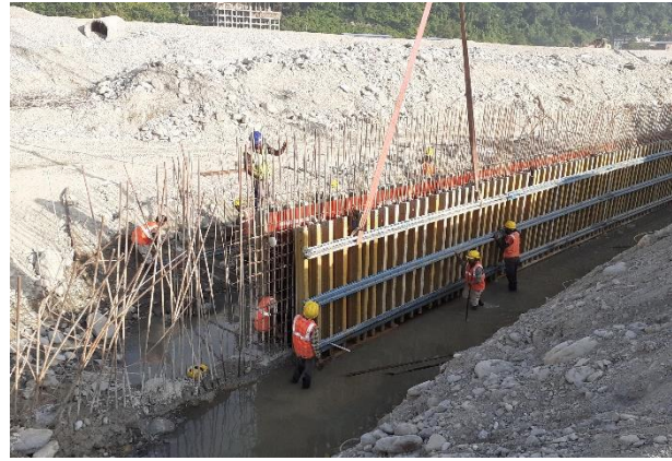
Preparing for formwork installation
