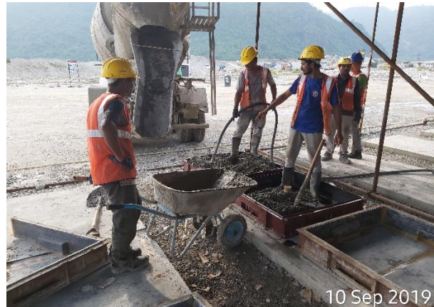
Concrete pouring into formwork
