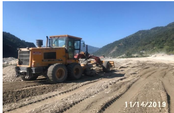
Dumping and Spreading for earth filling work
