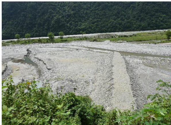
Spurs at end termination at PART-8
