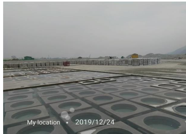
Curing of the precast blocks for 28 days
