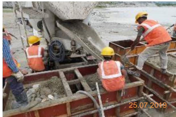
Concreting the blocks
