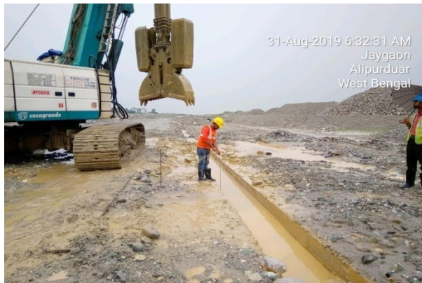
Sounding check after excavation works
