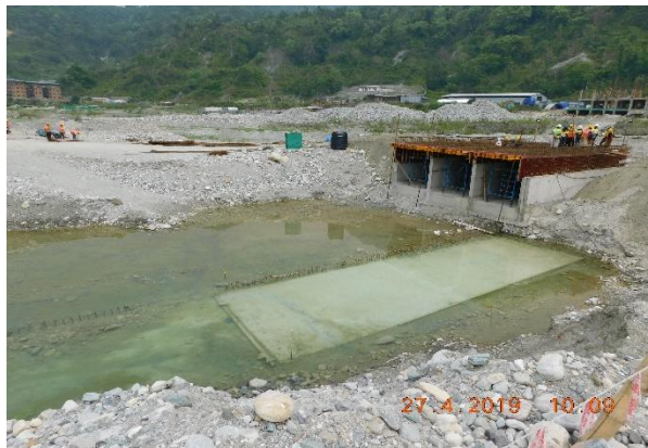
Concreted ducted structures and dewatering after heavy rainfall
