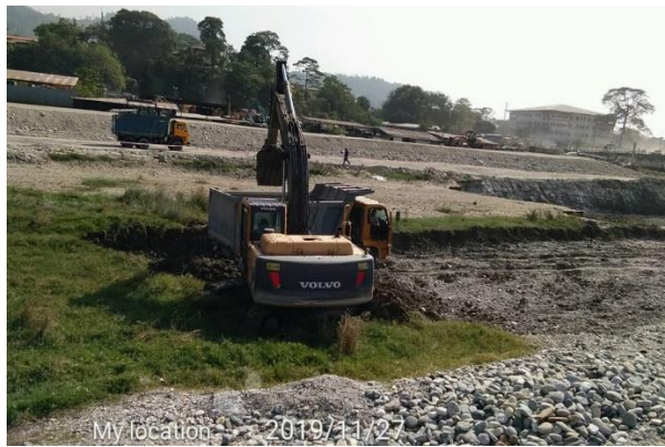
Removal of unsuitable materials before earth filling work
