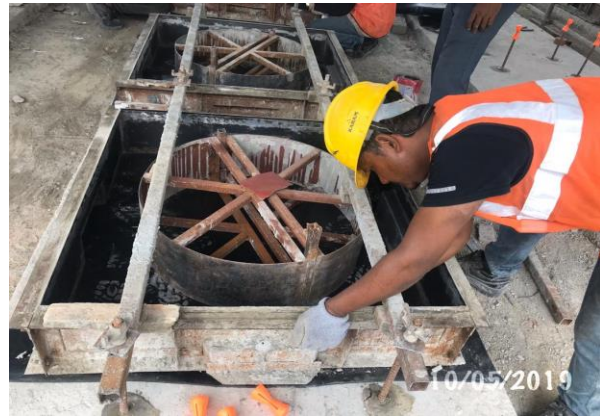
Formwork preparation for precast blocks
