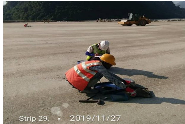
OMC test after compaction
