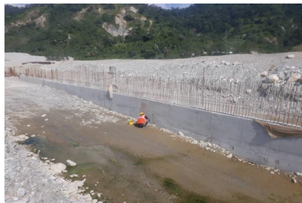
Concreted panel of cast in-situ wall
