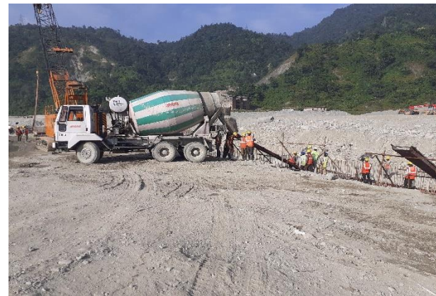
Concreting the cast in-situ wall panel
