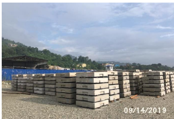
Stacking of precast blocks after curing
