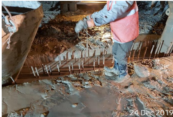
24 Dec 2019 Concreted panel top level check
