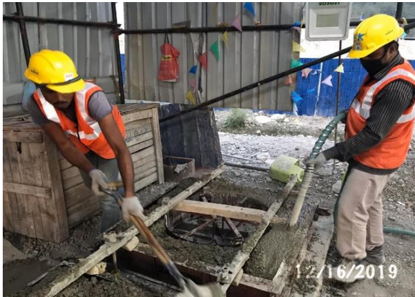
Concrete pouring into formwork
