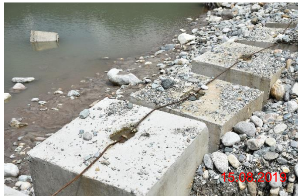
Concrete blocks at scourage area
