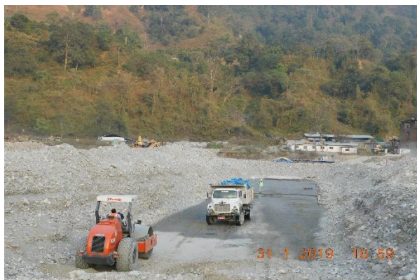
Excavations and PCC laying for the outfall structures
