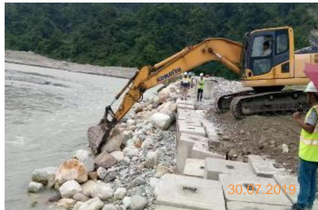
Placing of concreted blocks for river protection
