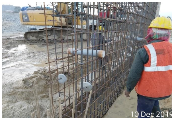
PVC Weep holes installation
