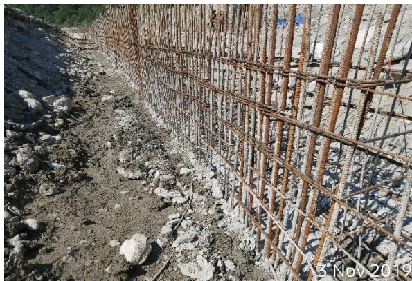
13 Nov 2019 Rebar arrangement for cast in situ wall
