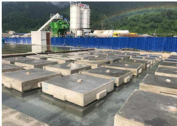
Curing of the precast blocks for 28 days
