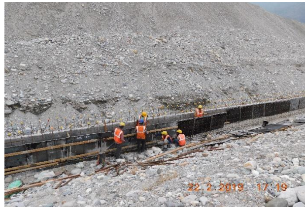
Guide wall work: Excavations and formwork preparations for vertical wall
