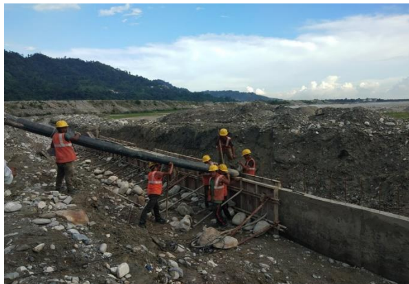
Guide wall work: Concreting the vertical wall
