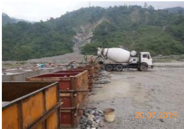
Mould preparation for concrete cube blocks
