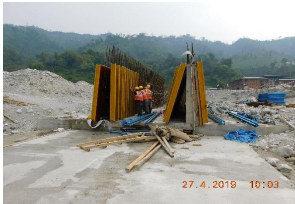
Formwork installations, concreting and removal of formworks
