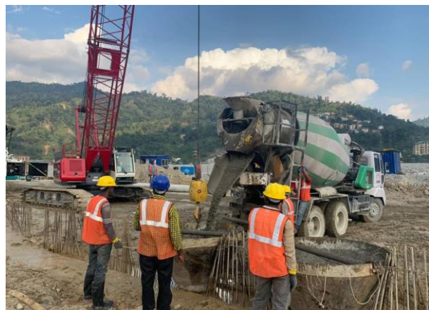
Concreting the Diaphragm wall panel
