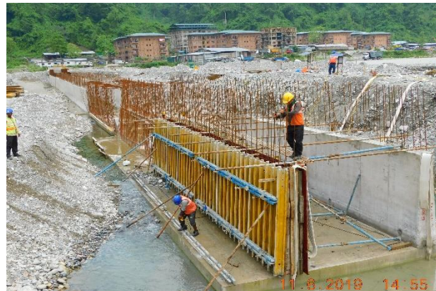
Formwork installations, concreting and removal of formworks
