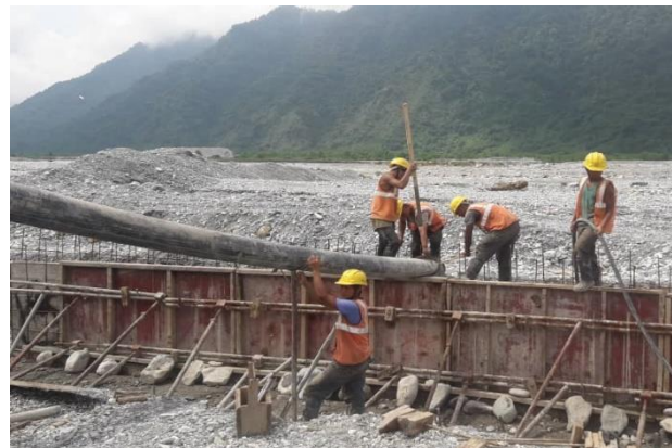
Guide wall work: Concreting the vertical wall
