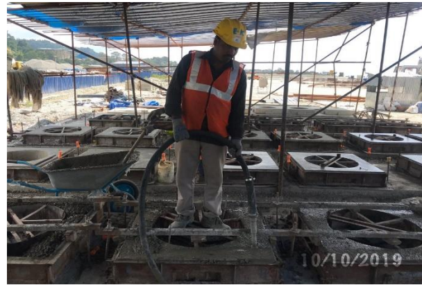
Using vibrators for compaction of concrete
