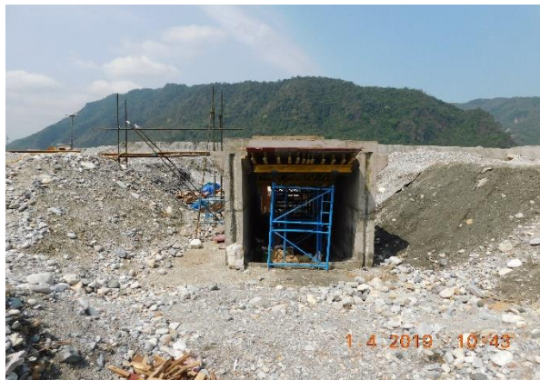
Concreted ducted portion of the Outfall structures
