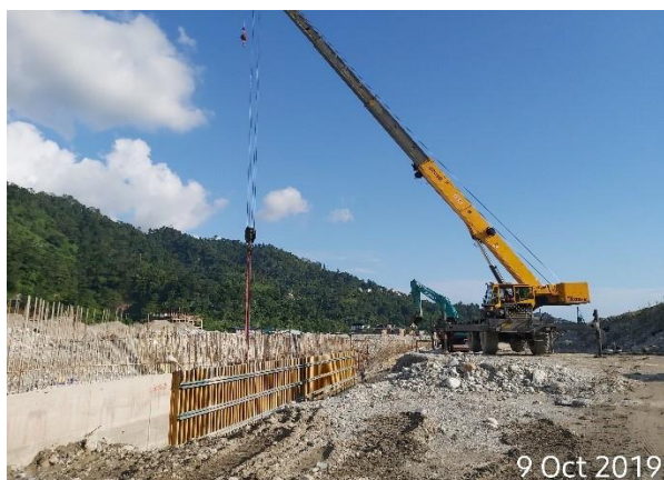
Removal of formwork for concreted panel of cast in-situ wall
