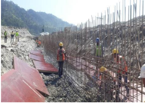
Preparing for formwork installation
