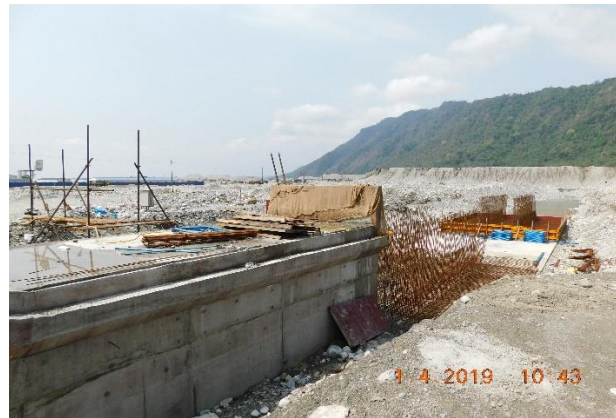
Concreted ducted portion of the Outfall structures
