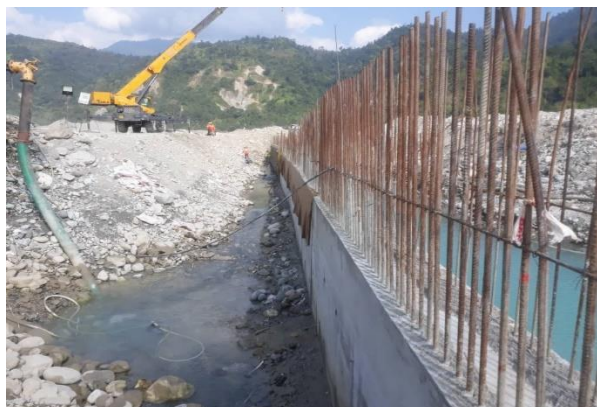
Concreted panel of cast in-situ wall
