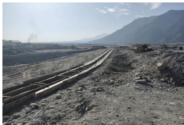
Guide wall concreted
