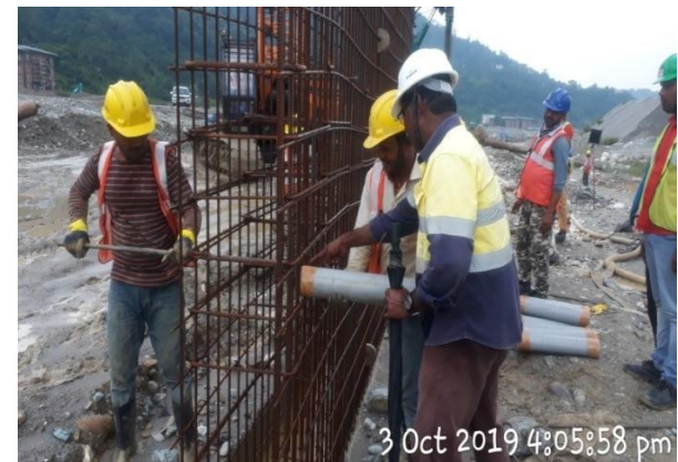
PVC Weep holes installation
