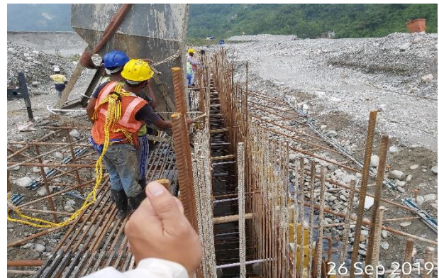
Concreting for cast-in situ
