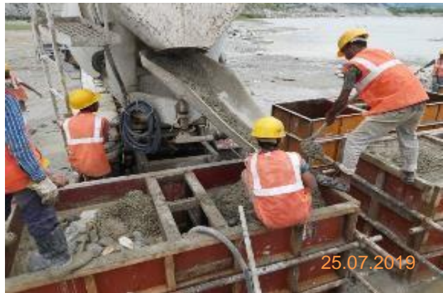
Concreting the blocks
