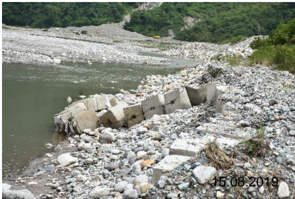
Concrete blocks washed away during a heavy rain fall
