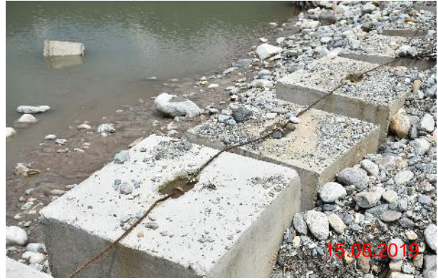
Concrete blocks at scourage area
