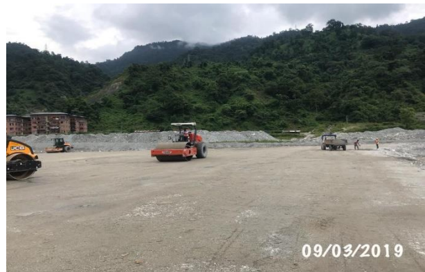
Compacting the earth fill
