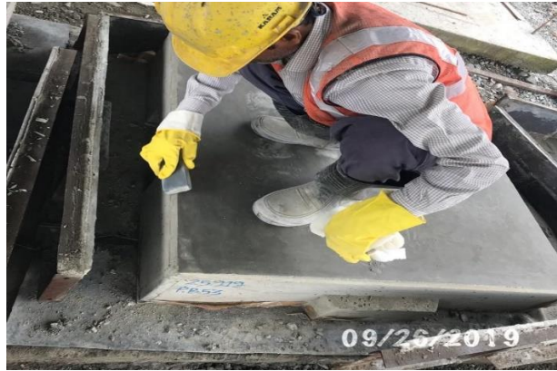
Mould removal for precast block
