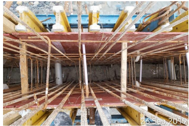
Formwork preparation for cast-in situ wall
