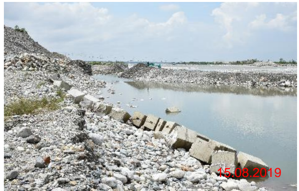
Concrete blocks washed away during a heavy rain fall
