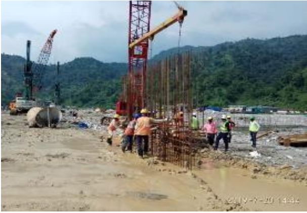
Rebar cage installation
