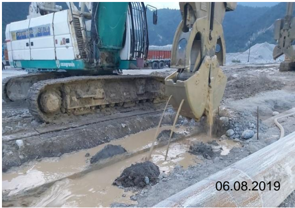
Excavations for D-wall panel
