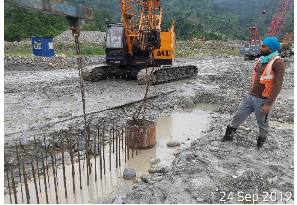
Rebar cage installation
