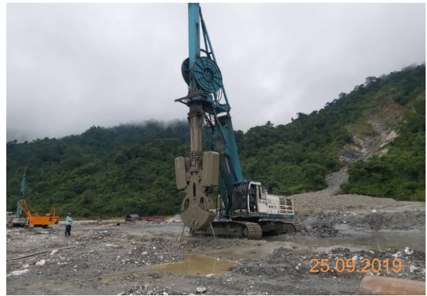
Excavations for D-wall panel
