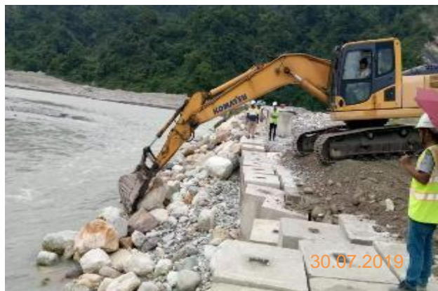
Placing of concreted blocks for river protection
