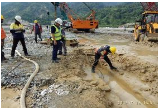
Sounding check: excavations depth
