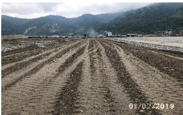
Spreading for earth filling work
