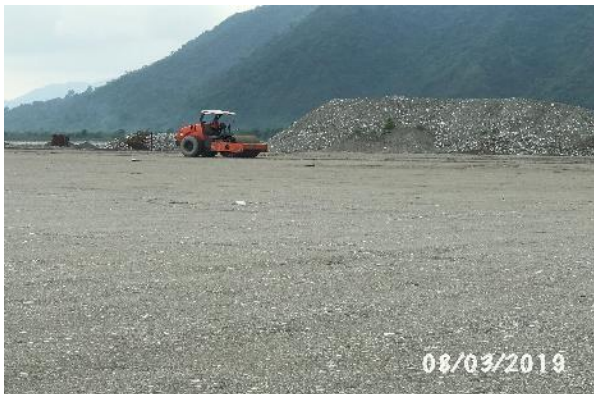
Compacting the earth fill
