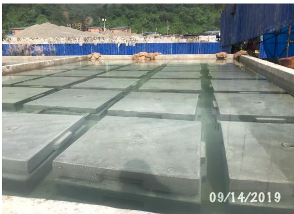
Curing of blocks in curing pond
