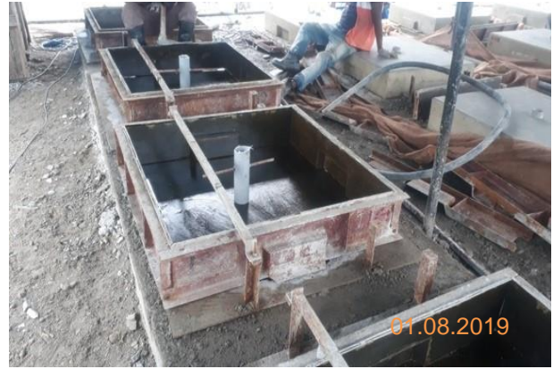
Mould preparation
