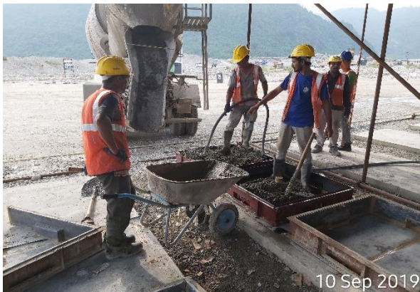
Concrete pouring into mould
