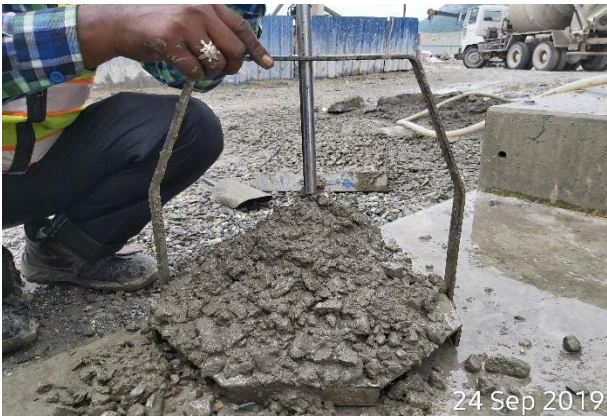
Slump test before concreting the panel
