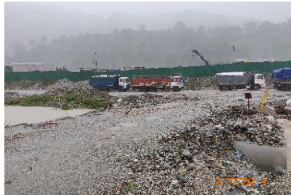
Trucks parked near the project boundary
