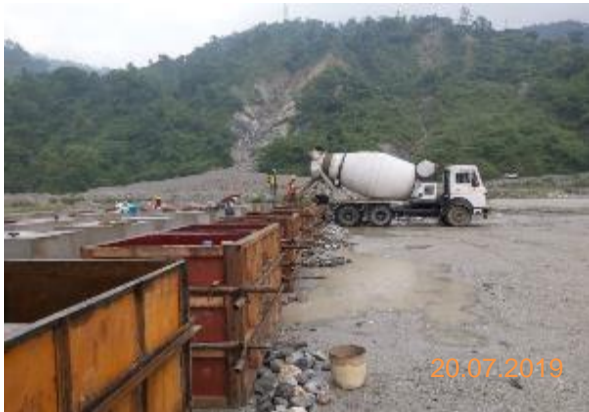
Mould preparation for concrete cube blocks
