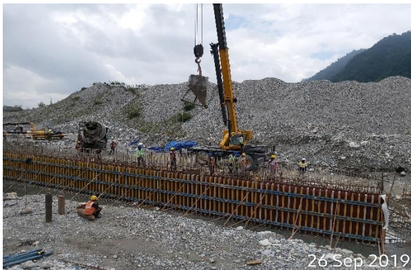
Concreting for cast-in situ
