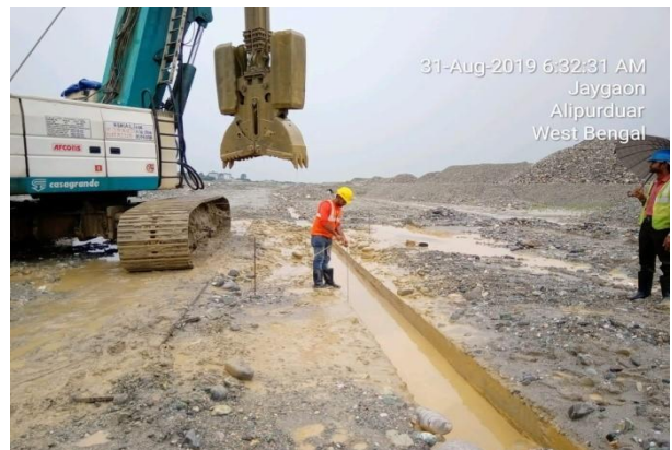
Sounding check: excavations depth
