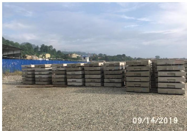
Stacking after 28 days of curing
