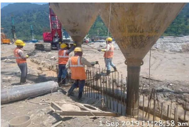
Concreting the D-Wall panel
