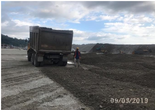
Dumping for earth filling work
