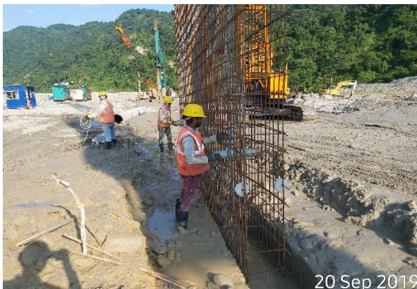
PVC Weep holes installation
