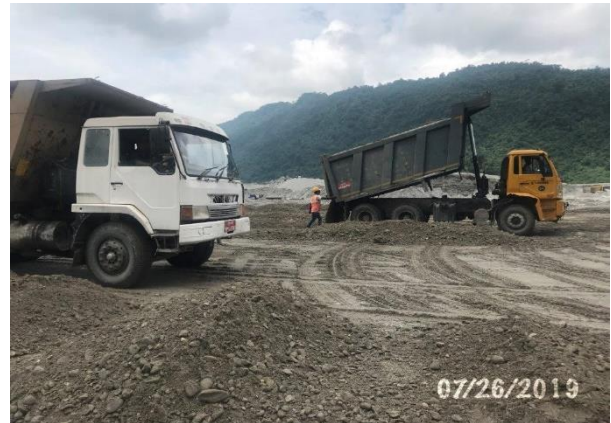
Dumping for earth filling work
