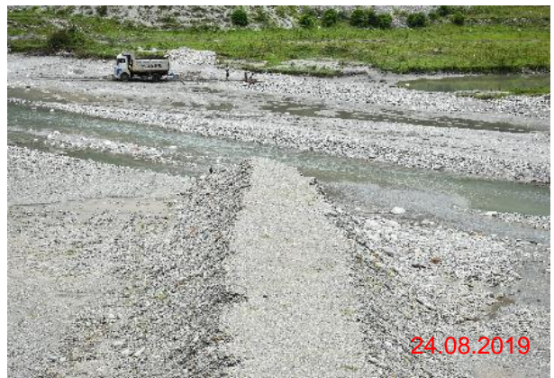
Spurs at end termination at PART-8
