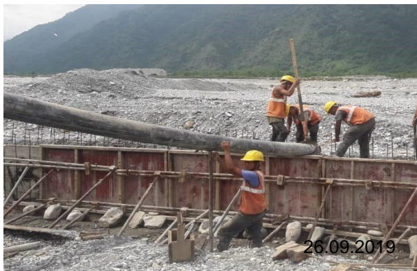
Guide wall: formwork preparation and concreting
