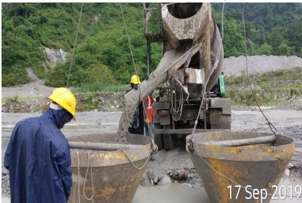
Concreting the D-Wall panel
