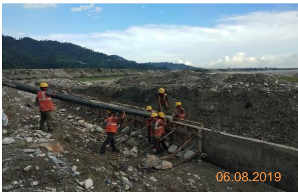
Guide wall: concreting and formwork removal
