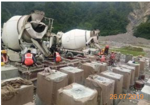
Curing the blocks at site
