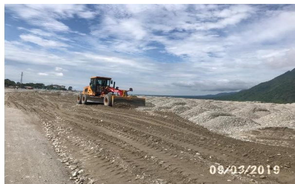
Spreading for earth filling work
