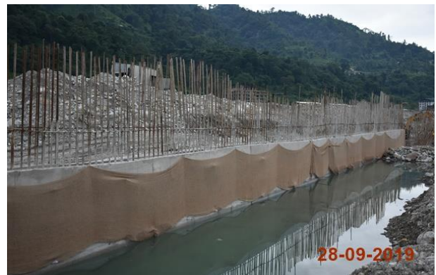
Concreted panel of cast in situ wall
