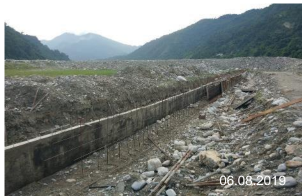
Guide wall: concreting and formwork removal
