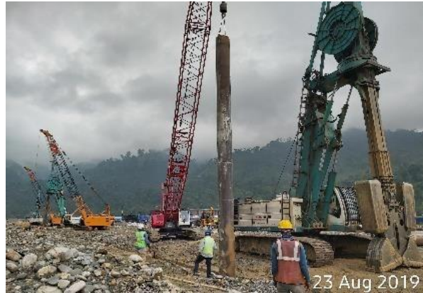
Stop end installation
