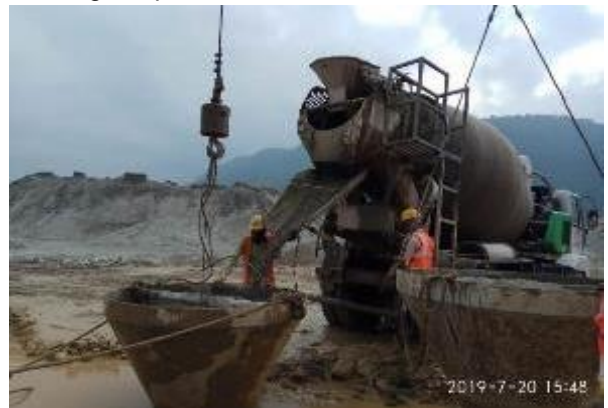
Concreting the D-Wall panel
