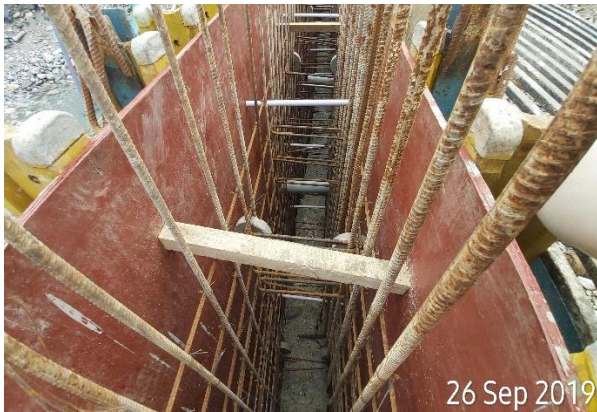
Formwork preparation for cast-in situ wall
