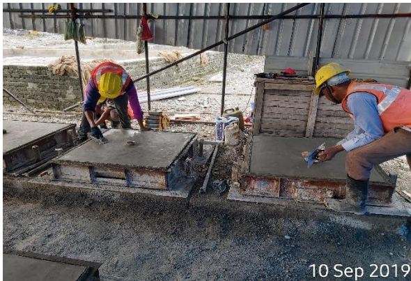
Precast blocks finishing works
