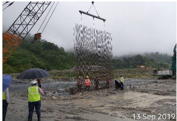
Rebar cage checking and lowering
