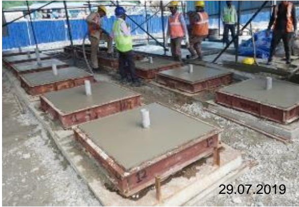
Precast blocks finishing works
