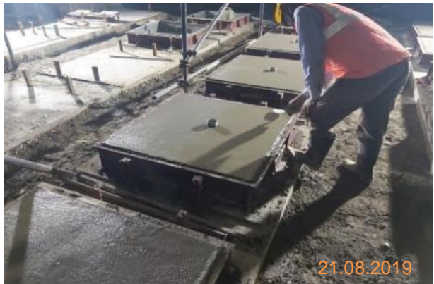
Precast blocks finishing works
