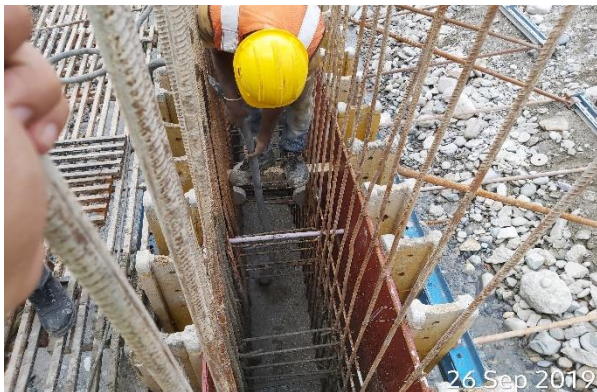
Compaction of concrete by vibrator for cast-in situ
