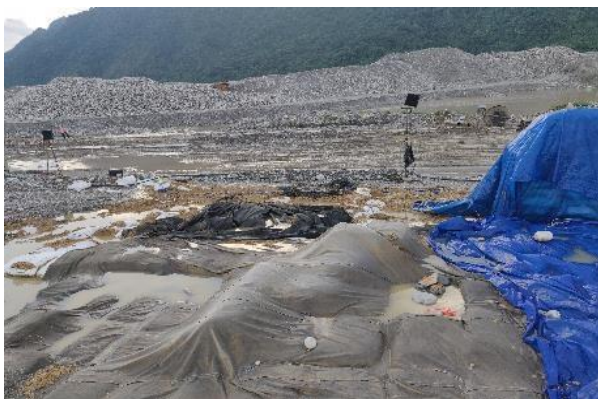
Bentonite covered at site with plastic sheet
