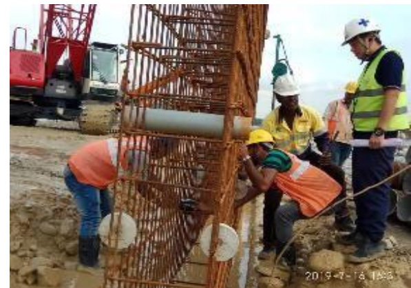
PVC Weep holes installation
