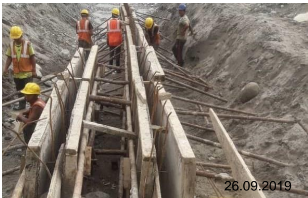
Guide wall: formwork preparation and concreting
