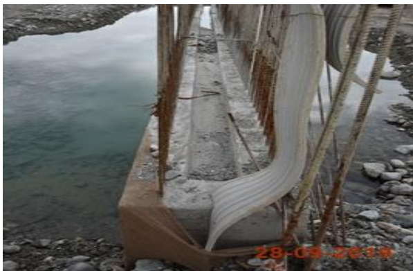
Concreted panel of cast in situ wall
