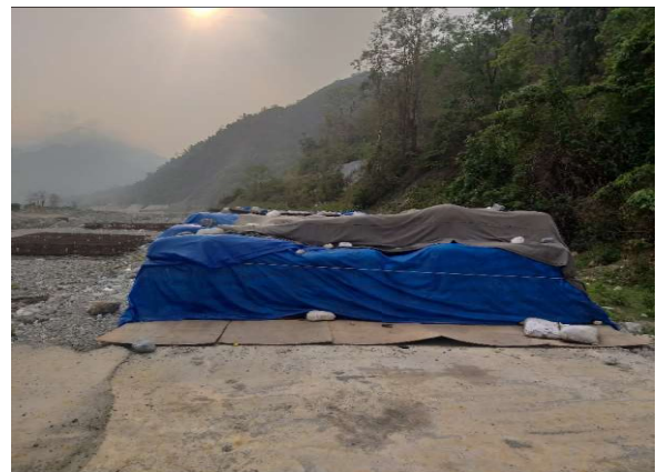
Bentonite sacks covered in Tarpaulin sheet and barricaded
