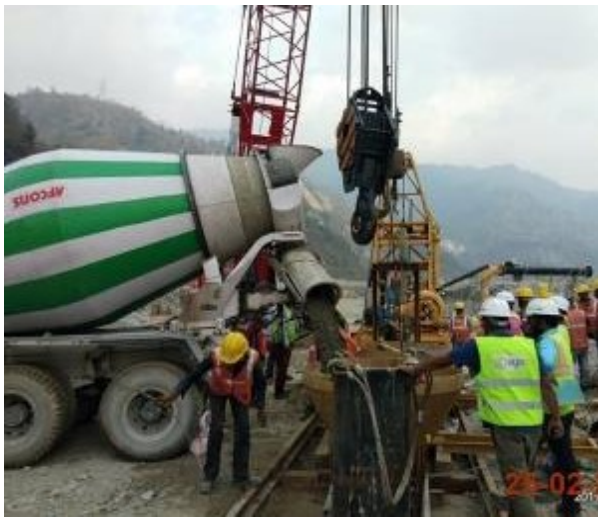
Diaphragm wall-Concrete casting
