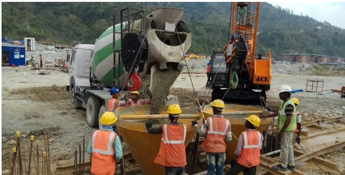
Diaphragm wall-Concrete casting
