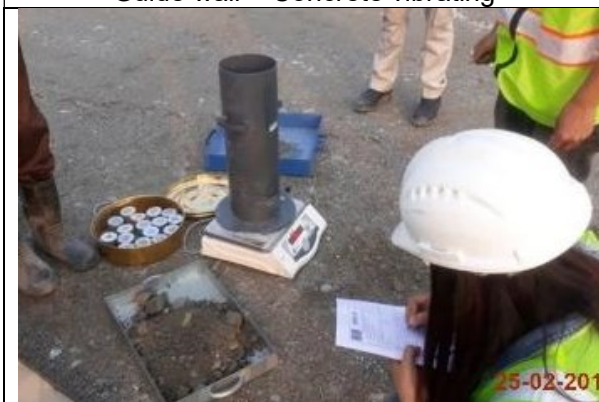
Filling works – Field density test
