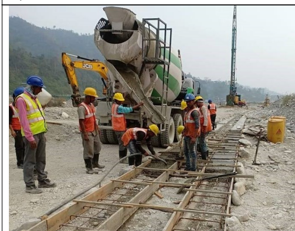
Guide wall – Concrete vibrating
