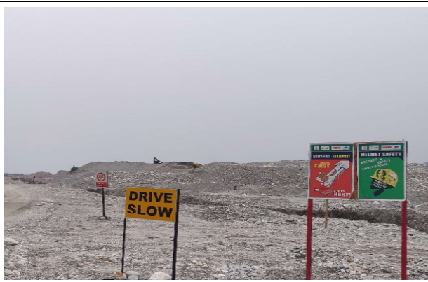
Safety Sign boards at works site diversion
