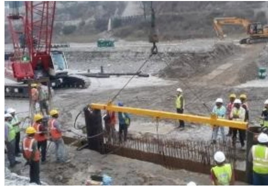
Diaphragm wall- Rebarcage installation
