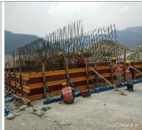
Open outfall n°02 – Steel rebar installation
