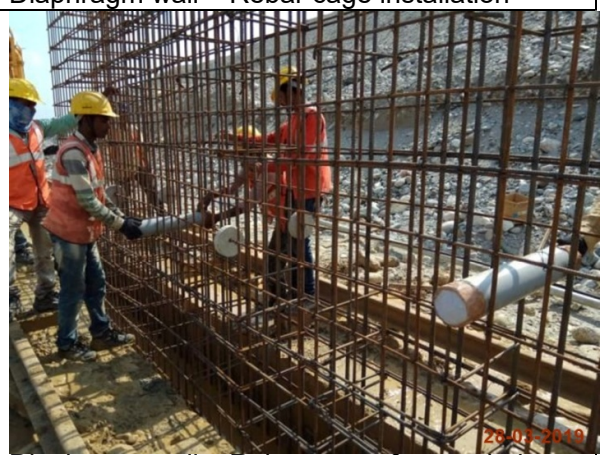
Diaphragm wall – Rebar cage & weep hole
