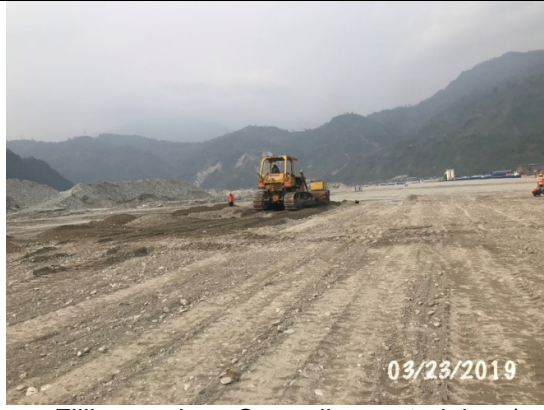
Filling works – Spreading materials w/ bulldozer
