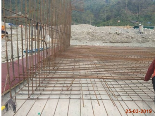
Open outfall n03 – Steel rebar installation
