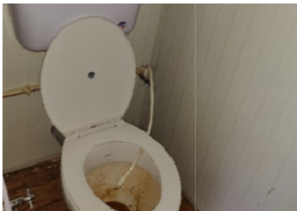
Dysfunctional toilet at site
