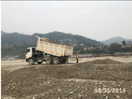
Filling works – Unloading materials
