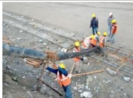
Guide wall – Day concrete cast
