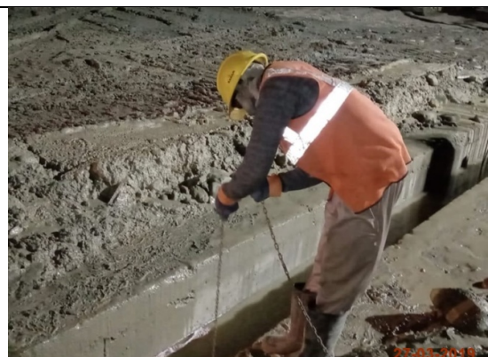
wall – Excavation depth measurement
