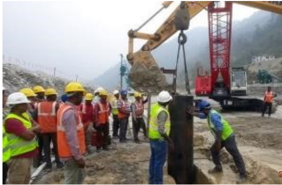
Diaphragm wall-Stop ends installation
