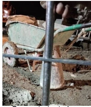
Concrete test slump
