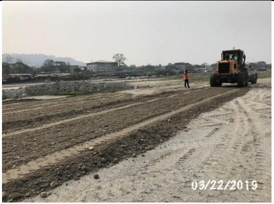
Filling works – Spreading materials w/ grader
