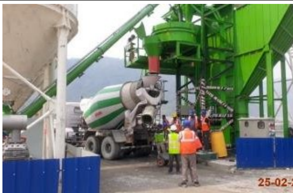
Batching Plant – Concrete production
