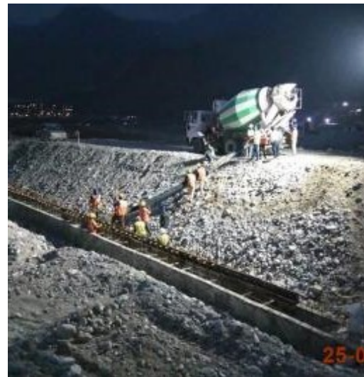
Guide wall- Night concrete cast
