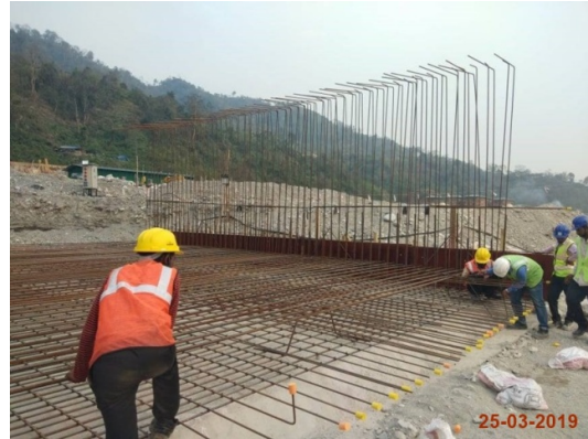
Filling works – Unloading materials
