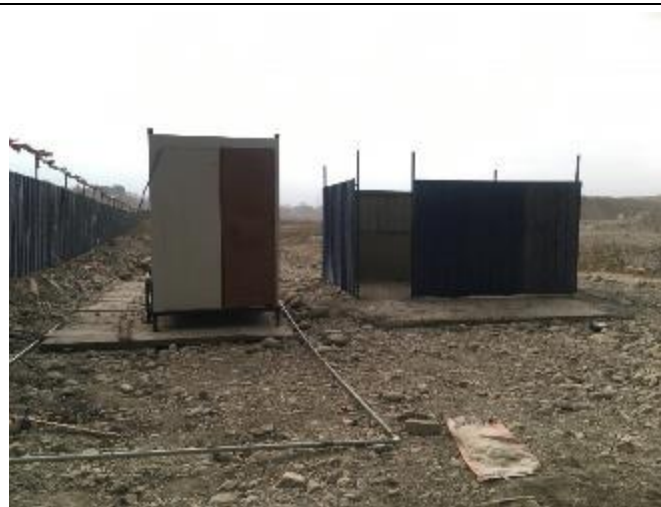
Photograph 9: Toilets and bath rooms at site
