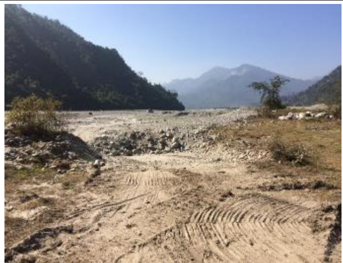
Photograph 8: Bund Creation and blocking access to Stop Car Washing in River
