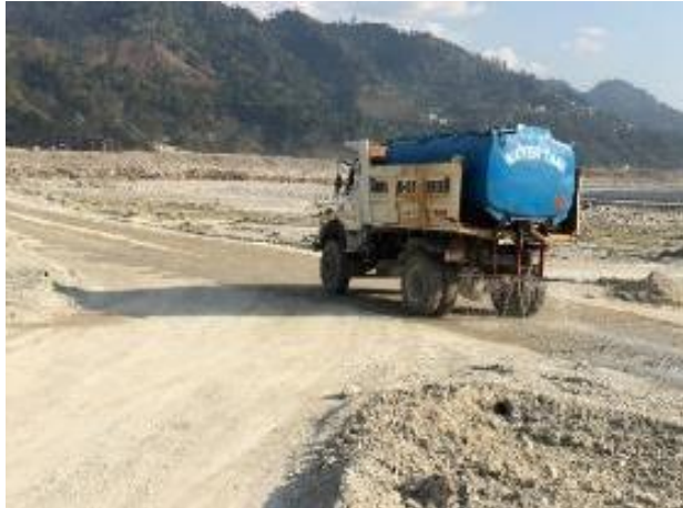
Photograph 1: Water Sprinkling carried out for the Dust Suppression
