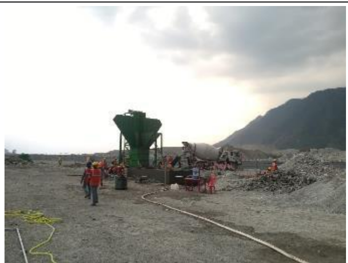
Photograph 10: Workers using PPE
