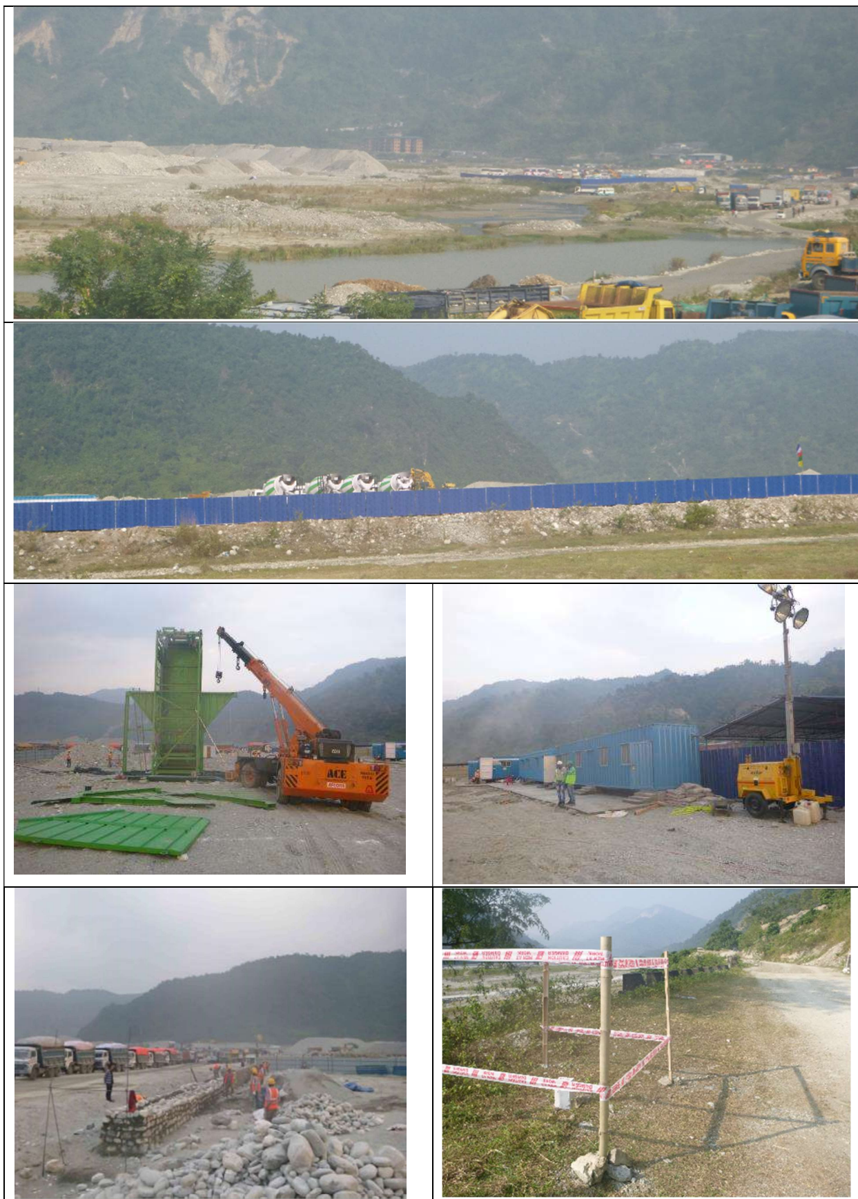
Figure D.1-2: Contractor's mobilization – 30 November 2018
