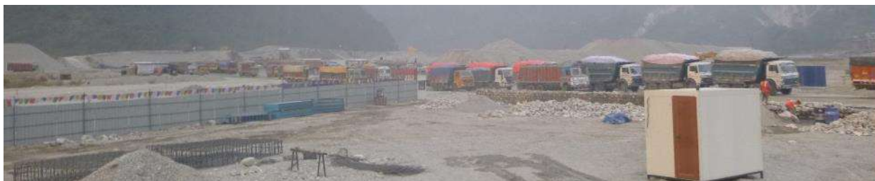
Figure E.2-3: Traffic through camp site and external vehicles parked
