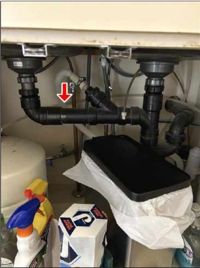
10.8 Item 1(Picture) drain slope
