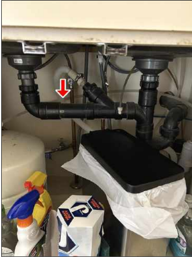
10.8 Item 1(Picture) drain slope
