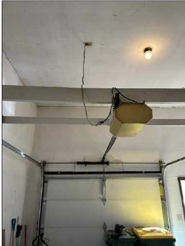
3.4 Item 1(Picture) older opener with extension cord wiring
