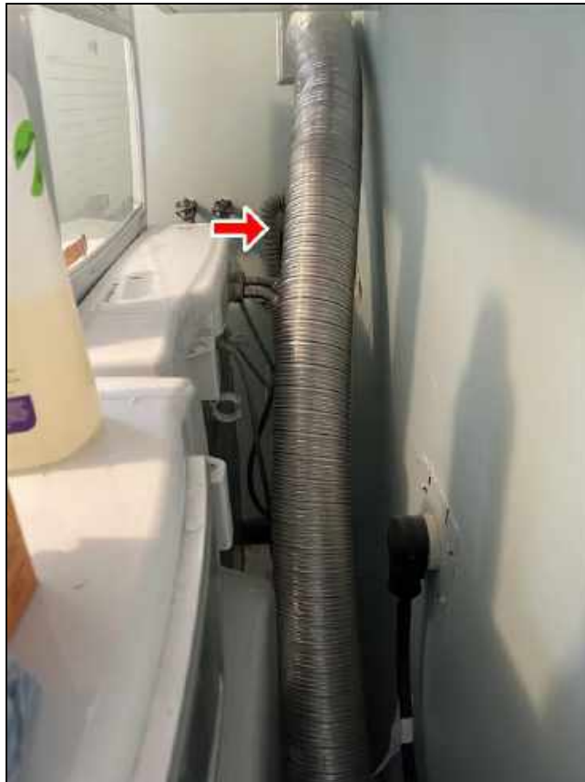
12.8 Item 1(Picture) gas dryer vent
