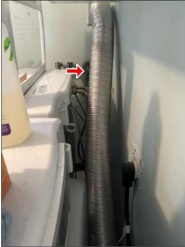
12.8 Item 1(Picture) gas dryer vent
