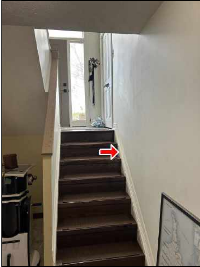
13.9 Item 1(Picture) missing railing
