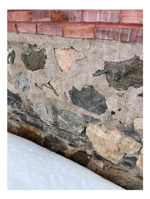
Concrete has been added at the right wall; it is completely stable.
