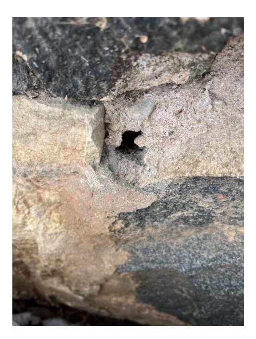
This work includes openings at the stone concrete junction, at the right foundation.
