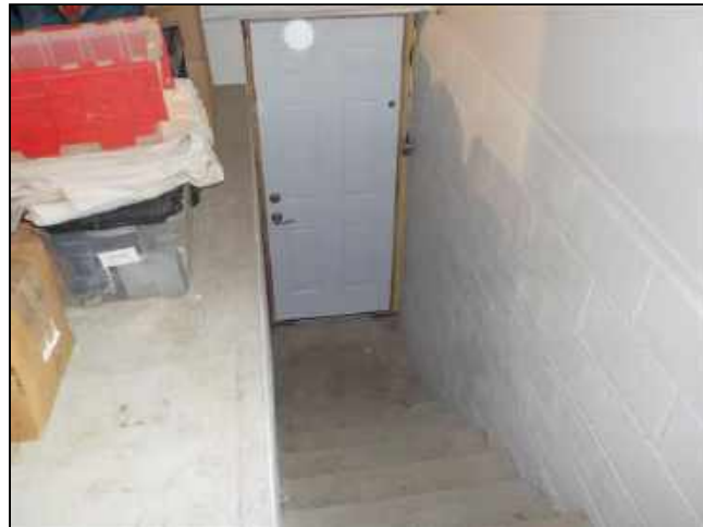
3.10 Item 1(Picture) Missing railings
