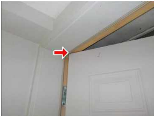
3.5 Item 1(Picture) Missing closer
