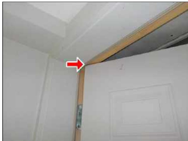
3.5 Item 1(Picture) Missing closer
