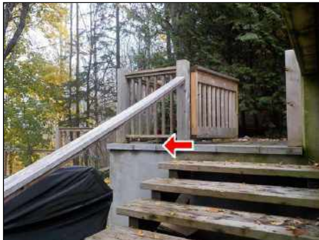
1.11 Item 1(Picture) Stair railings
