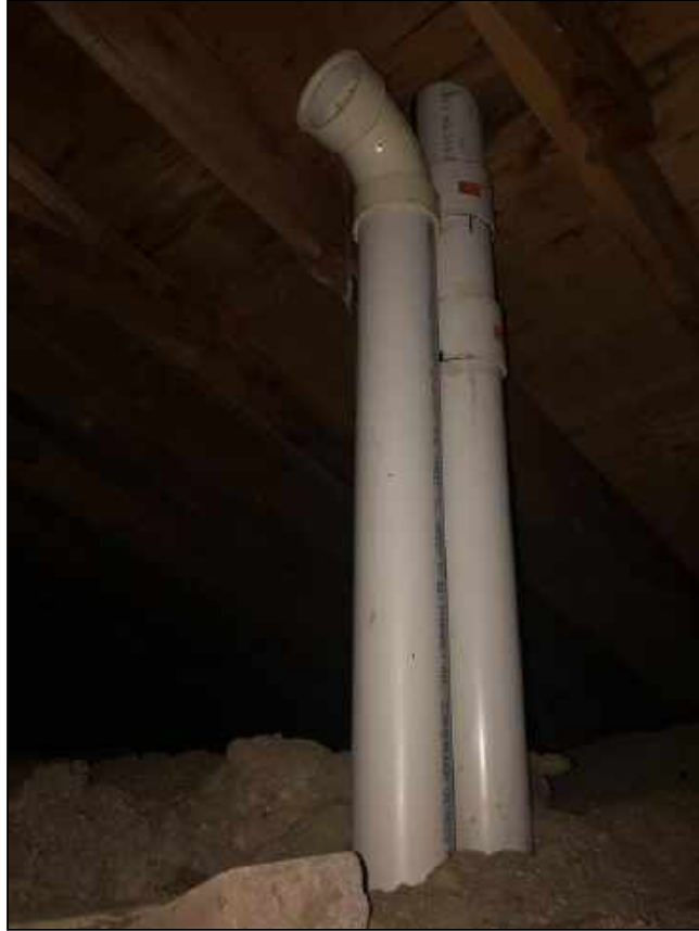
8.2 Item 1(Picture) Venting conditions
