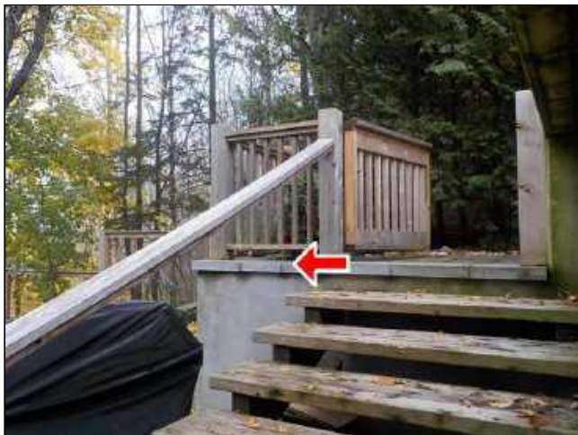
1.11 Item 1(Picture) Stair railings
