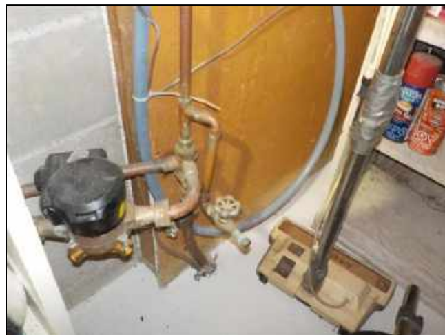
6.0 Item 1(Picture) Main shut off
