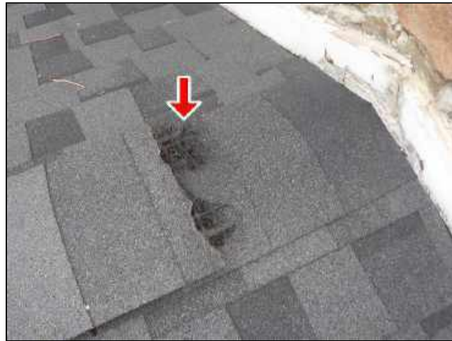
2.1 Item 1(Picture) Damaged ridge vent
