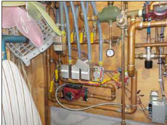
8.4 Item 1(Picture) Zoned controls and distribution piping
