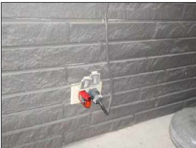
1.7 Item 1(Picture) Standard outlet and light wiring
