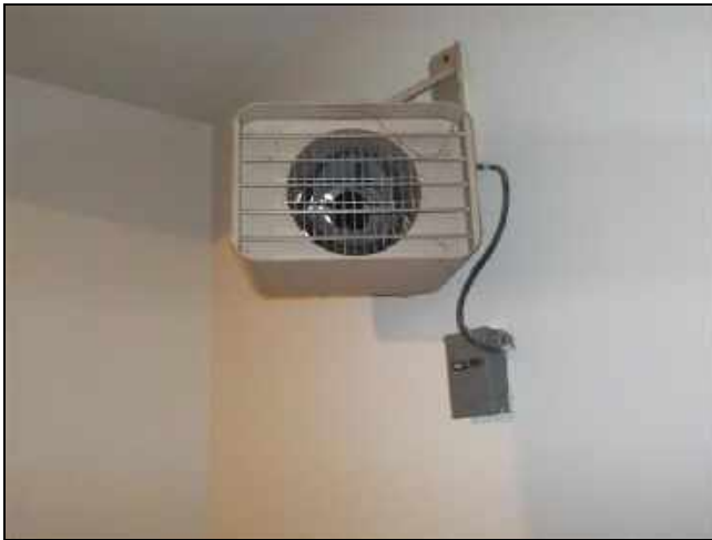
3.9 Item 1(Picture) Obsolete heater
