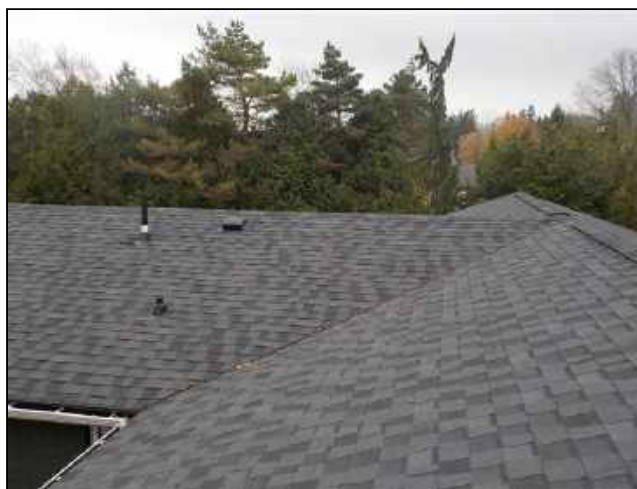
2.0 Item 1(Picture) Roof conditions
