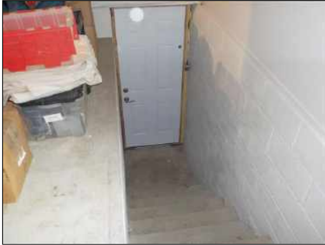
3.10 Item 1(Picture) Missing railings
