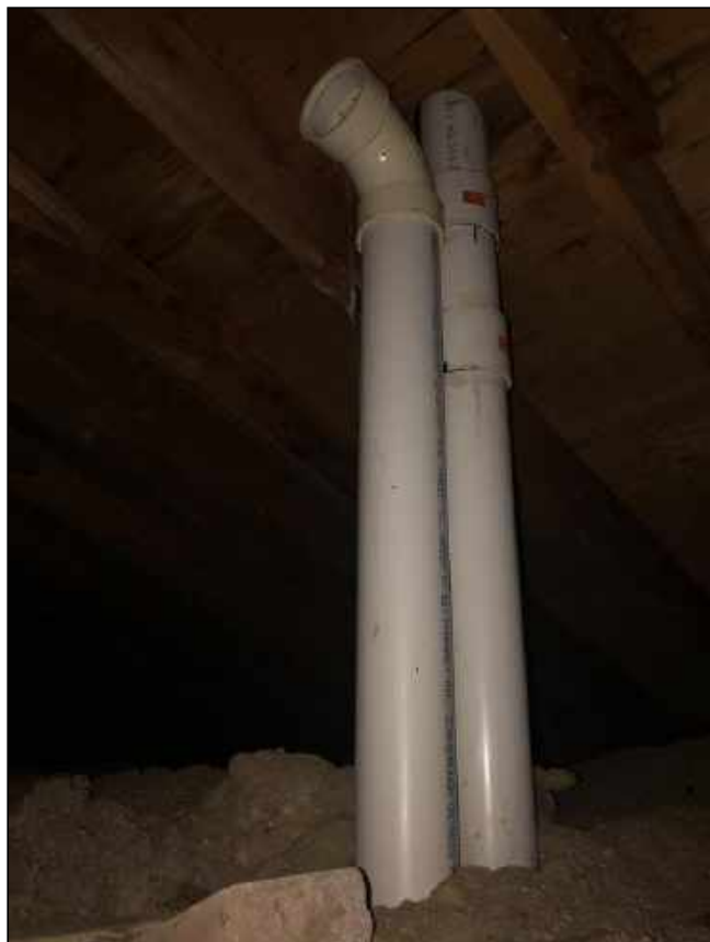
8.2 Item 1(Picture) Venting conditions
