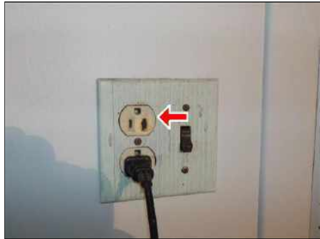
3.9 Item 2(Picture) Damaged outlet
