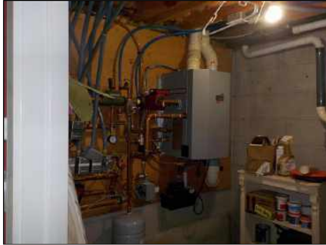
8.0 Item 1(Picture) Direct vent gas boiler
