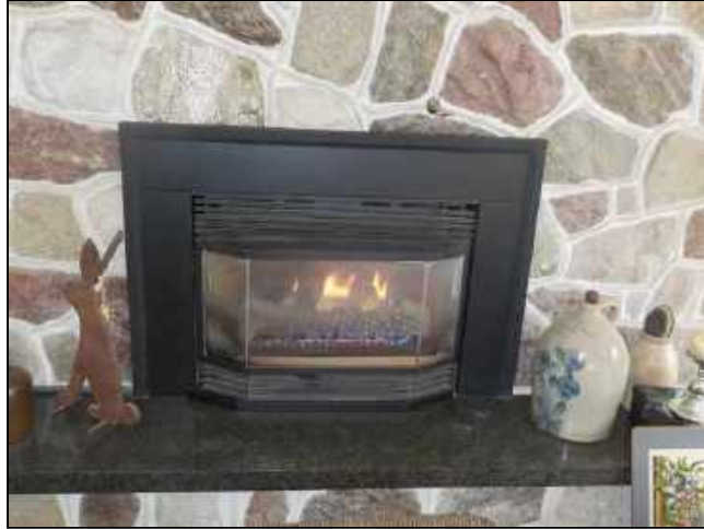
13.8 Item 1(Picture) Gas fireplace
