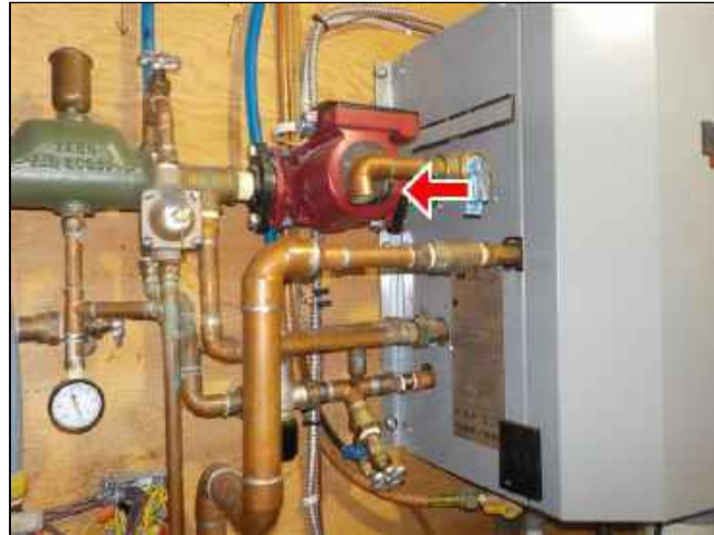
9.4 Item 1(Picture) Missing extension pipe
