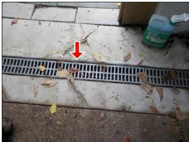
1.10 Item 2(Picture) Trench drain
