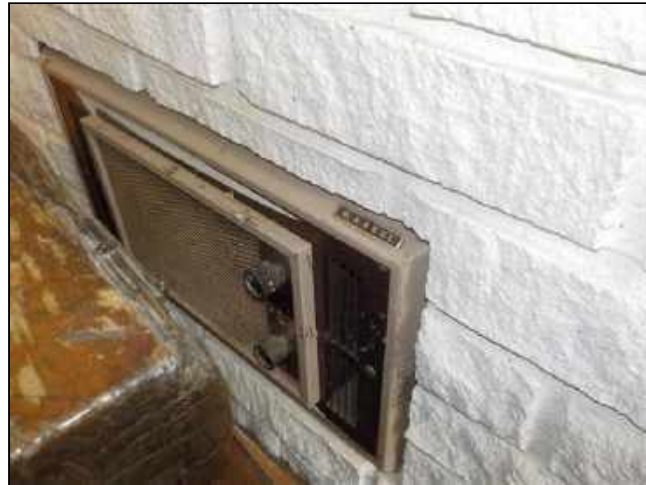
10.3 Item 1(Picture) Obsolete electric heater
