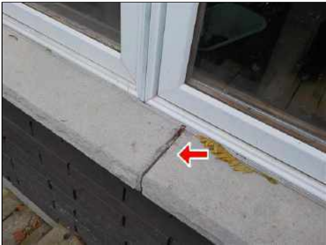
1.4 Item 1(Picture) Sill mortar condition
