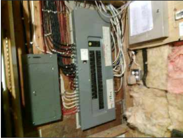
7.2 Item 1(Picture) Main panel and junction box
