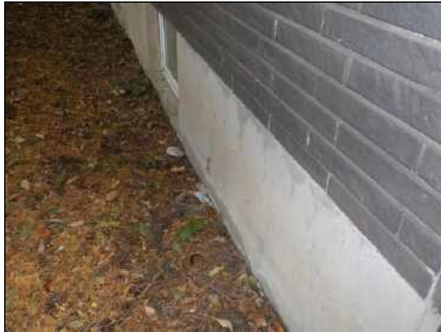
1.10 Item 1(Picture) Low drainage area
