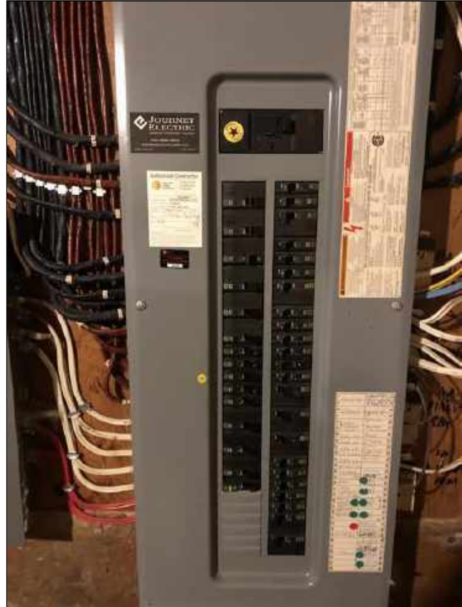
7.2 Item 2(Picture) Inspection tag
