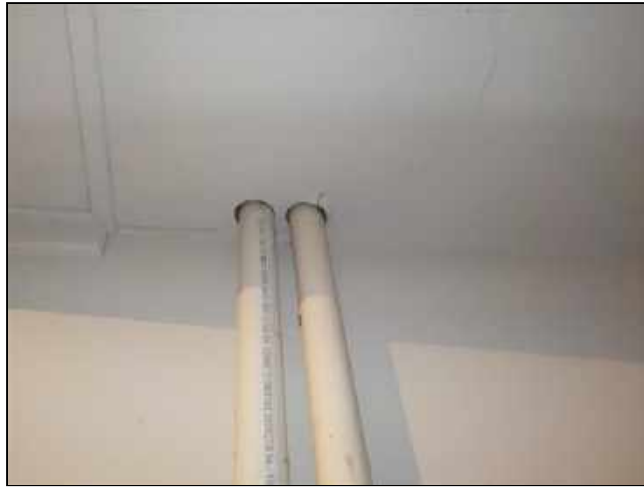
3.10 Item 2(Picture) Vent pipes
