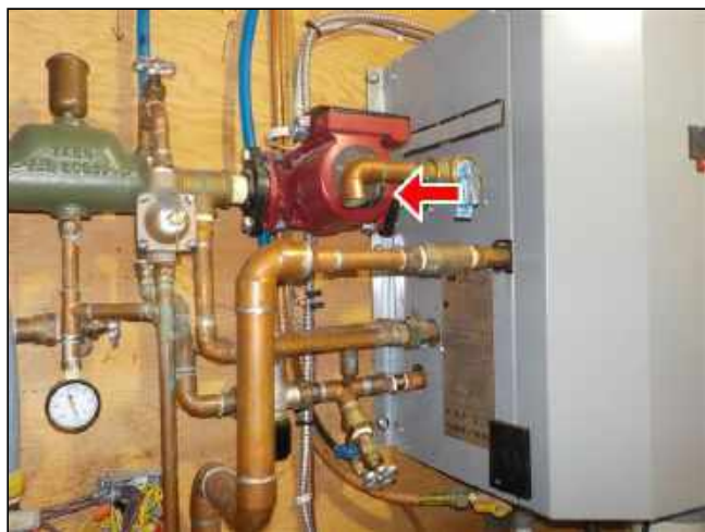
9.4 Item 1(Picture) Missing extension pipe
