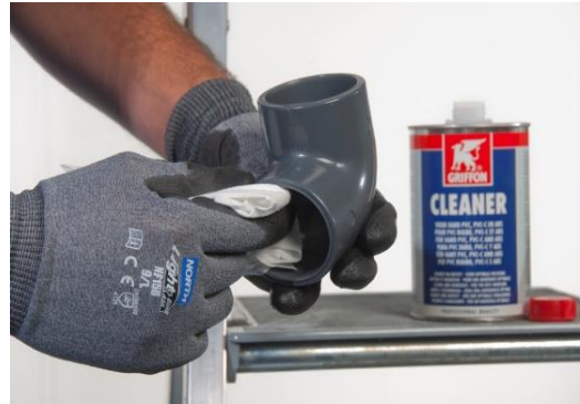
Step 5: Clean the fitting
