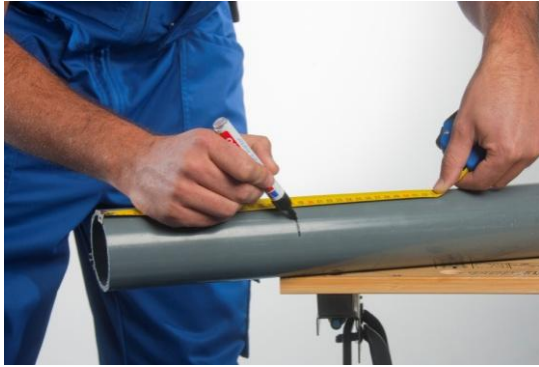
Step 1: Mark the pipe
