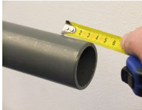
And mark pipe
