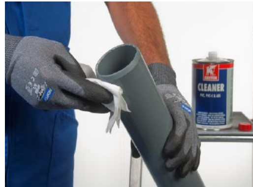
Clean the pipe end
