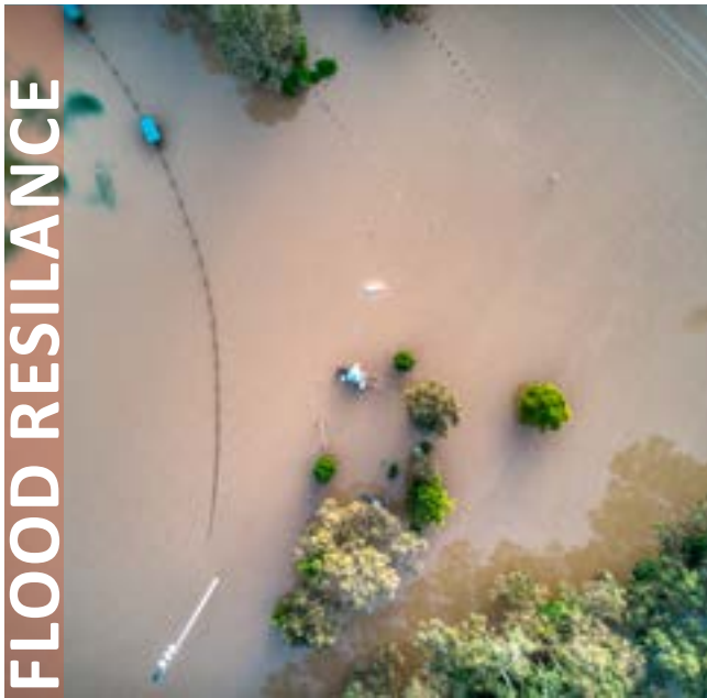
Unanderra Station Upgrade To address flooding from extreme rainfall, lifts were raised above maximum flood levels and a new drainage system was installed to manage excess water and mitigate future flood impacts.
