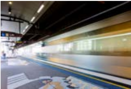
LEADERSHIP IN RAIL INFRASTRUCTURE
